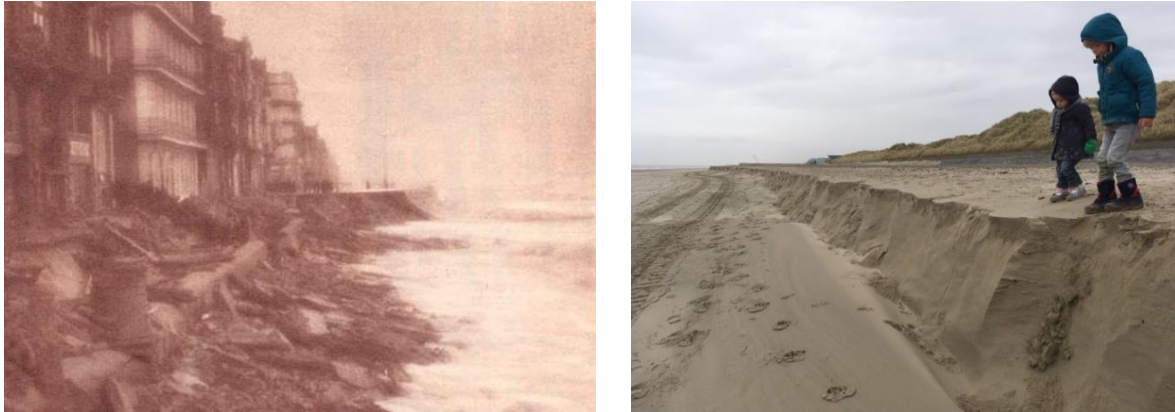
Figure B-8. Near failure of the Belgium coastal defence at Knokke-Heist in 1953 (Source: Le Patriote Illustré) and, more recent, formation of cliffs in 2013 (Source: T. Verwaest)
