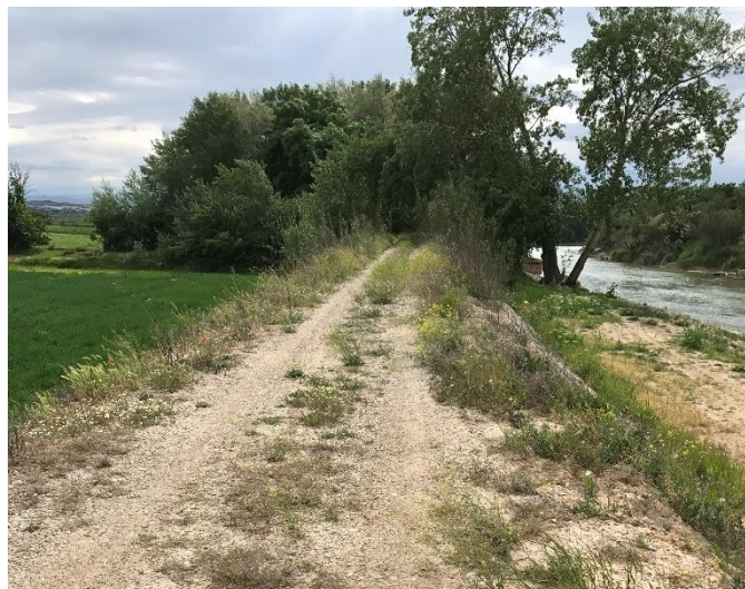
Figure ES-2. Levee segment in the Ebro river in Novillas (Zaragoza). Source: MITECO (Spanish Ministry for Ecological Transition).
