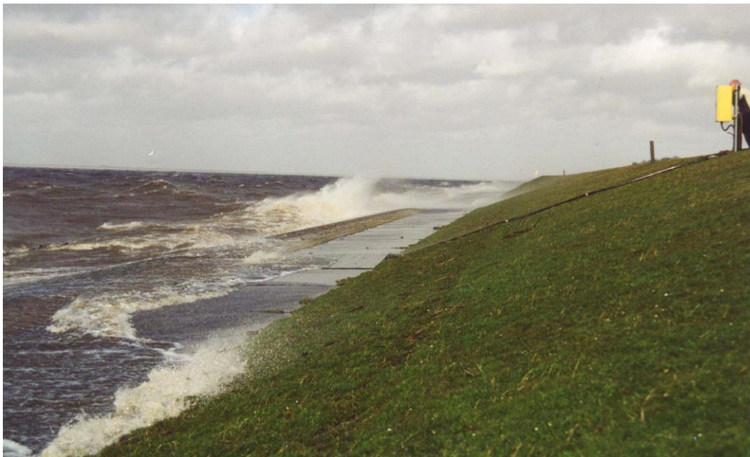
Figure NL-1: Rural lake-side levee during storm, with waves well above 1 metre (rubble-stone waterline berm and lower half of slope with placed stone partly submerged).
