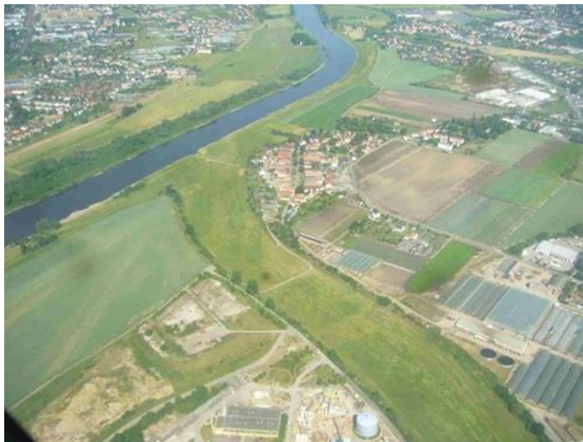
Figure D-2 Levees at the floodplains of the Elbe river (federal waterway) and on both sides of the flood bypass channel downstream the city of Dresden at Kaditz Village in the centre of the picture (photograph: R. Pohl)
