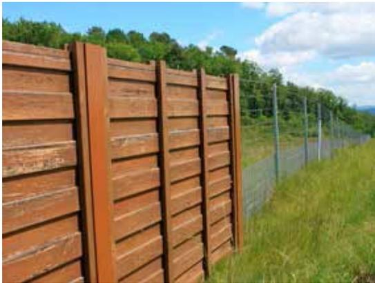
Figure 2.5. Screens on crossings must be in perfect continuity with the road perimeter fence. Photo: C. Rosell.
