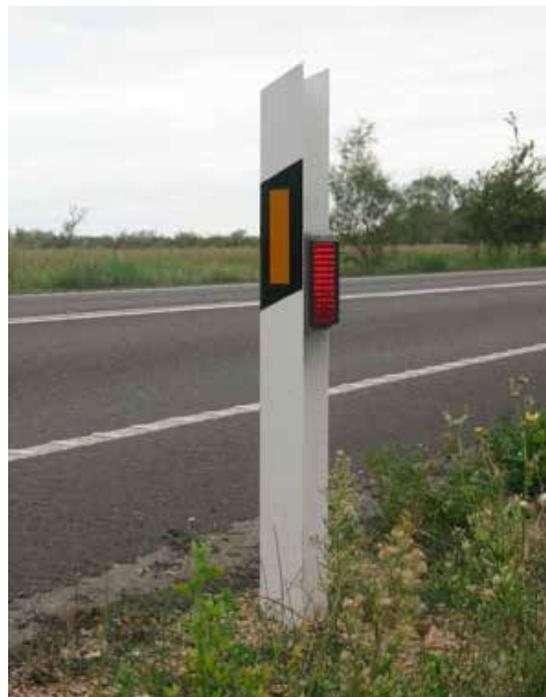
Figure 18.2. Various models of reflectors are available to project headlight beams into the natural surroundings of roads. These systems require frequent maintenance and have short-term effectiveness. Photos: C. Rosell.
