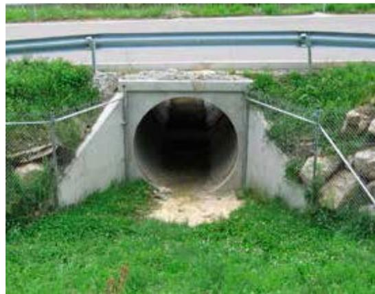
Figure 12.6. Correctly installed perimeter fencing. Photo: M. Fernández-Bou.
