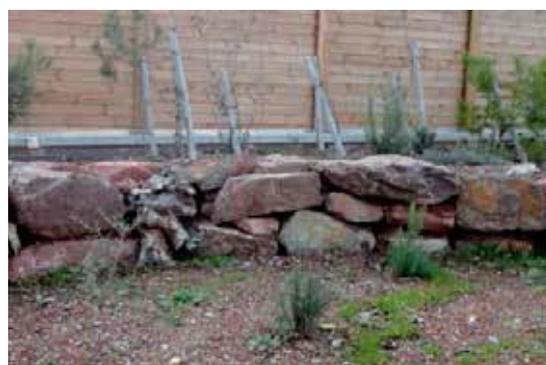
Figure 1.9. Low dry wall constructions provide micro-habitats for small animals along the edge of the ecoduct. Photo: S. Vanpee - IRSTEA.
