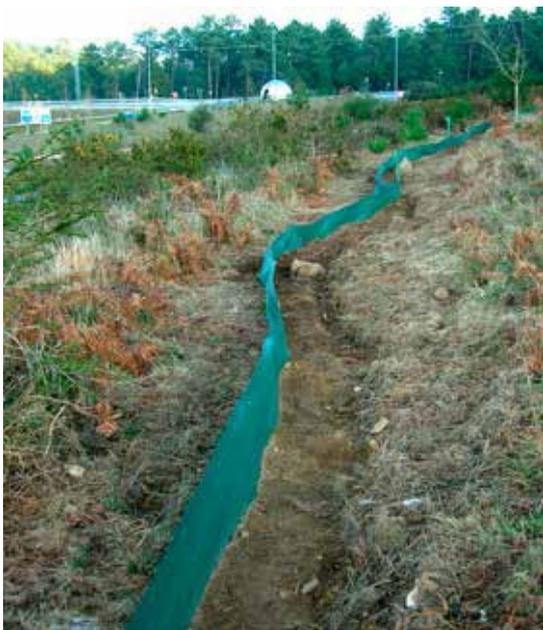
Figure 11.8. Temporary barrier combined with collection buckets. Photo: Environment Office, University of Vigo.
