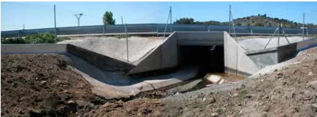
Figure 11.7. Fence leading amphibians towards a wildlife crossing under construction. Photo: Javier Cantero.
