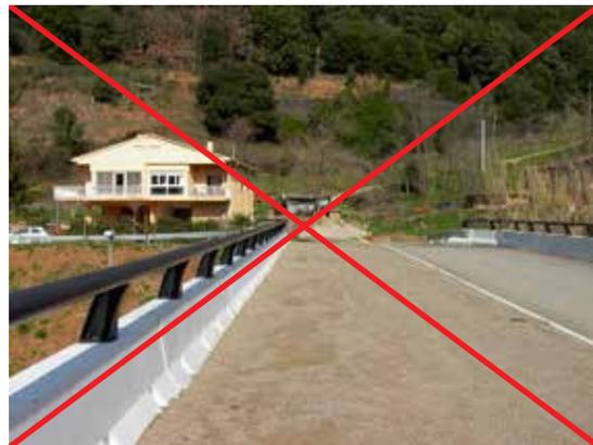
Figure 3.6. The lateral strip intended for use by wildlife should be covered with soil, not the gravel employed in this case. The location is also unsuitable due to the proximity of buildings. Photo: F. Navàs.
