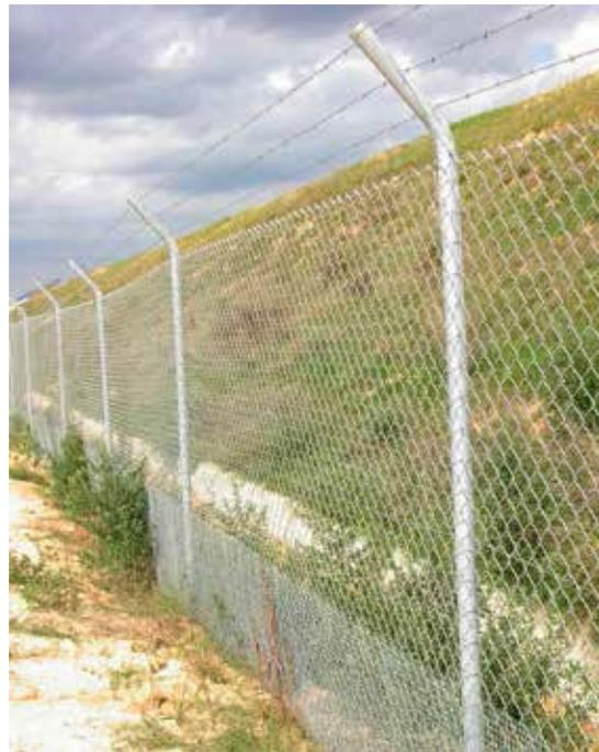
Figure 14.3. Fence combined with an outrigger to prevent deer from jumping over and base reinforcement for small vertebrates. Photo: M. Fernández Bou.
