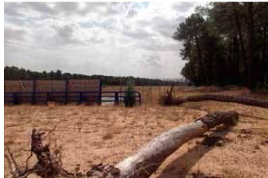
Figure 1.11. Two alternative systems using boulders and tree trunks to avoid vehicle movement across the ecodeuct. Another option is to install metal or timber barriers at a suitable height and signs prohibiting vehicular traffic.
