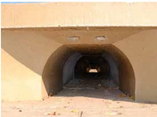
Figure 11.2. Interior of an amphibian crossing with a semi-circular section. The vertical walls and the flat base facilitate amphibian movement. Photo: M. Puky.
