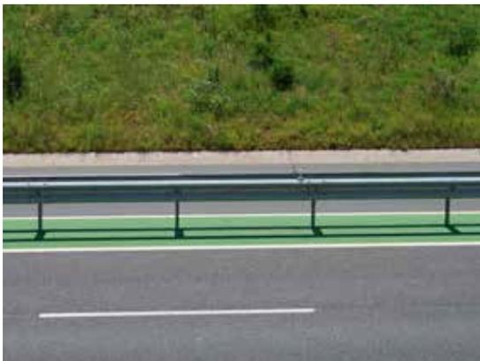
Figure 16.2. Unvegetated lane separation median strips. This may be appropriate on road sections where the proliferation of voles and other prey attract raptors and carnivores, increasing the roadkilling hazard. Photo: C. Rosell.
