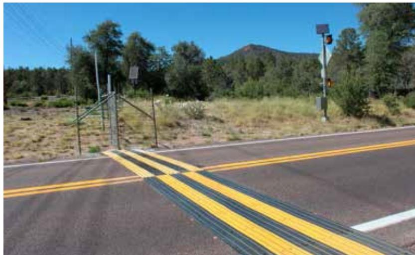
Figure 15.9. Electrified mat preventing animal entrance to a fenced main road via a paved access track. Photo: C. Rosell.
