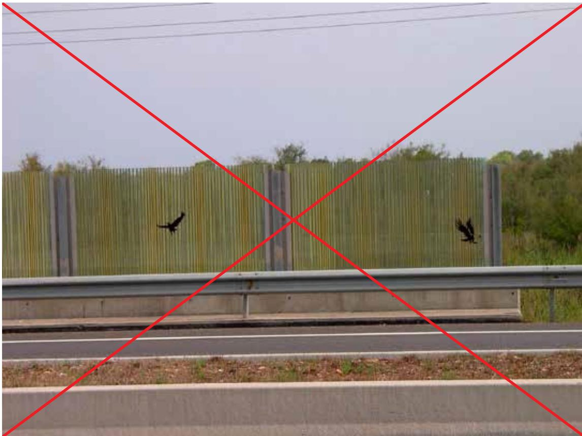
Figure 19.2. Transparent screen with silhouettes of birds of prey. This is ineffective for the prevention of bird collisions. Moreover, the vertical stripes do not stand out as they are the same colour as the surrounding vegetation. Photo: F. Navàs.
