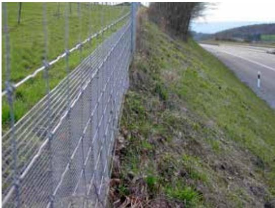
Figure 14.2. Reinforcement on the non-road side of conventional mesh. Photo: C. Rosell.
