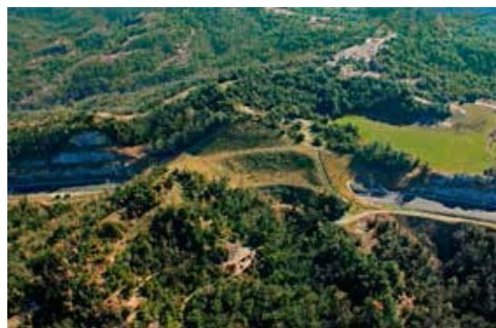
Figure 1.4. The ecoduct surface and access zones should have similar topographic profiles to the surrounding landscape. Photo: Minuartia.
