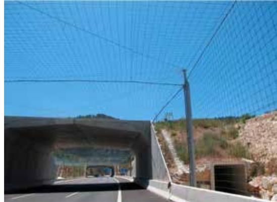
Figure 14.5. Polyamide net structure in a funnel shape to prevent bat collisions on a highway, with hitherto inconclusive results. Photo: M. Fernández Bou.
