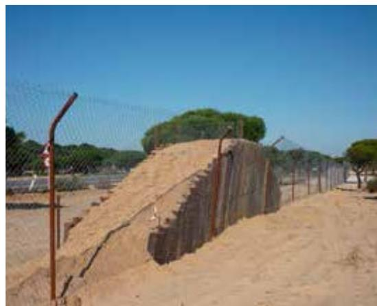
Figure 15.5. Escape ramp. On the left, viewed from the road side during the construction process, and right, viewed from the outside, once completed. Note that the fencing mesh has been removed at the top of the ramp to make it easier for animals to jump across. Photo: Public Works Agency. Government of Andalusia.
