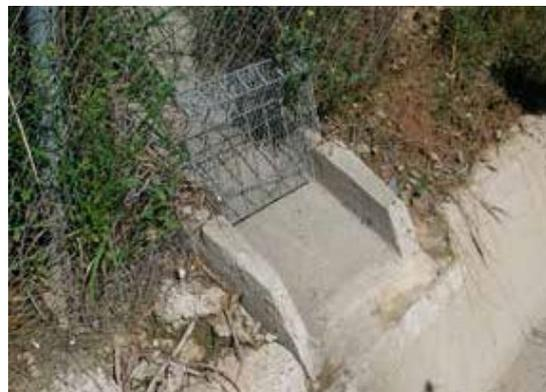
Figure 13.9. Two alternative systems to prevent animal passage at the interface between fences and roadside drains. Photos: Minuartia.
