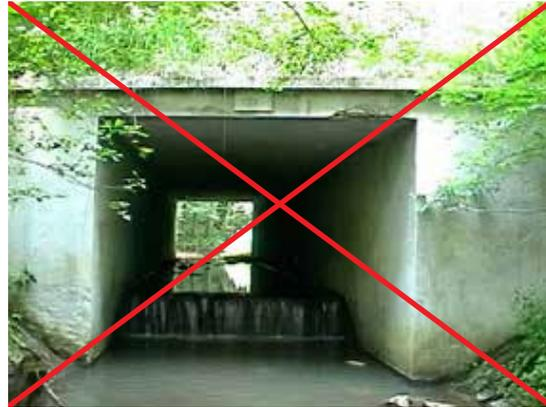
Figure 10.3. Step inside a culvert hindering the movement of aquatic fauna. Photo: J. Dufek.
