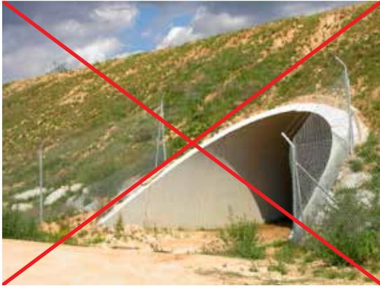
Figure 13.10. The fence should lead to the crossing, leaving no gaps that permit entrance to the embankment. Photo: C. Rosell.
