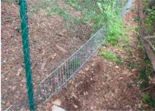
Figure 13.5. Wild boar reinforcement in a particularly troublesome section. Photo: Túnel Barcelona-Cadi.
