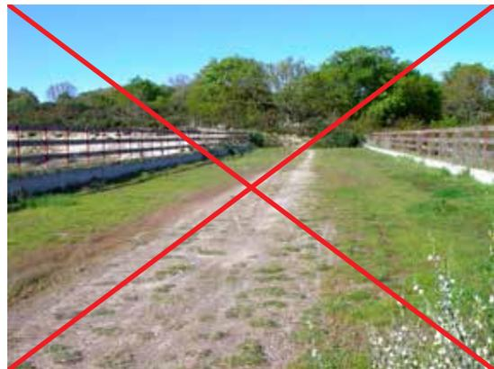
Figure 2.8. Motorized vehicle movements across an exclusive wildlife overpass and lateral screens that are not completely opaque. Photo: C. Rosell.
