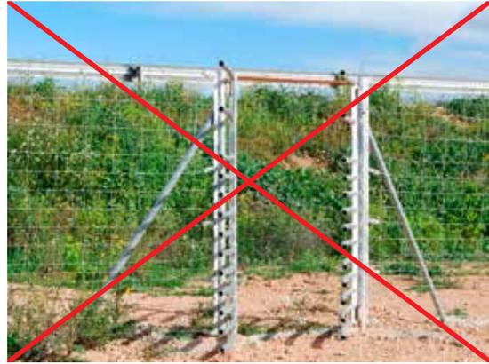
Figure 15.10. This ungulate escape gate can remain fully open, permitting free entrance by animals (and people) into the fenced area. Photos: F. Navàs.
