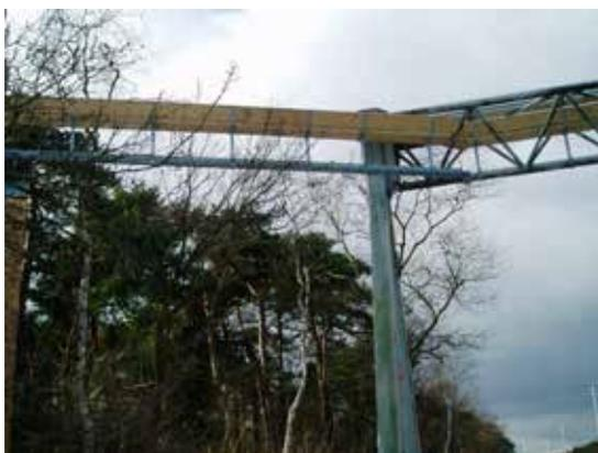
Figure 4.2. Timber platforms installed on a motorway sign post. Photo: H. Bekker.
