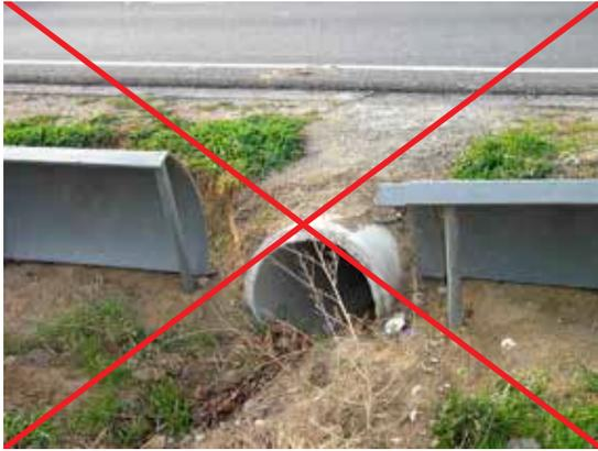
Figure 11.10. Maladjustment between guide structure and amphibian crossing entrance. Photo: C. Rosell.
