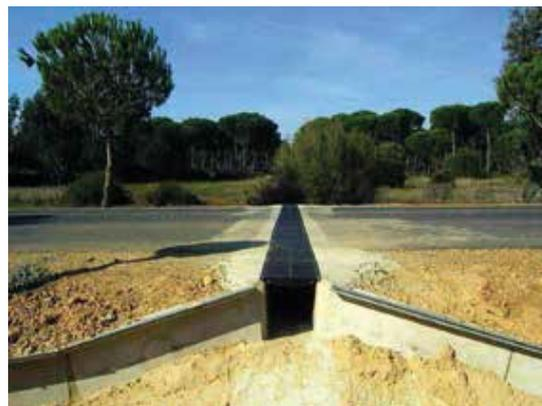
Figure 11.3. Amphibian crossing with funnel-shaped guide structure. Photo: GIASA.
