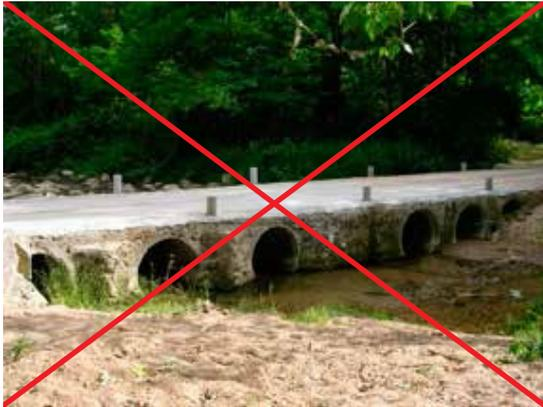
Figure 10.2. Drains located on a ford, hindering fish movements. Photo: F. Navàs.
