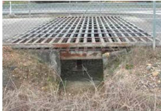
Figure 15.8. Cattle grid with a lateral escape aperture for small animals that might fall into the trench. Photo: Ministry of Public Works.
