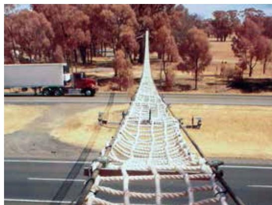
Figure 4.3. Mesh bridge crossing. In areas with a high fire risk, fire-resistant material must be used to prevent propagation. Photo: Kylie Soanes.
