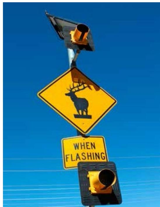
Figure 17.3. Flashing warning sign activated by animal detection sensors (ADS). Photo: C. Rosell.
