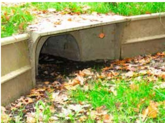
Figure 11.4. Amphibian crossing and prefab guide structure. Photo: M. Puky.
