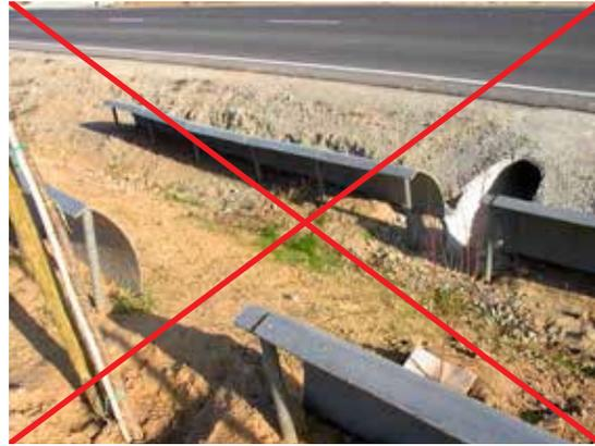
Figure 11.11. Discontinuity between different sections of the guide fences. Photo: F. Navàs.
