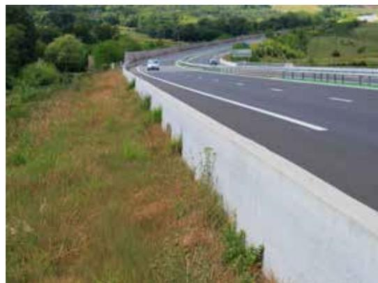
Figure 11.5. Opaque concrete fence, an optimum guide structure. Photo: C. Rosell.
