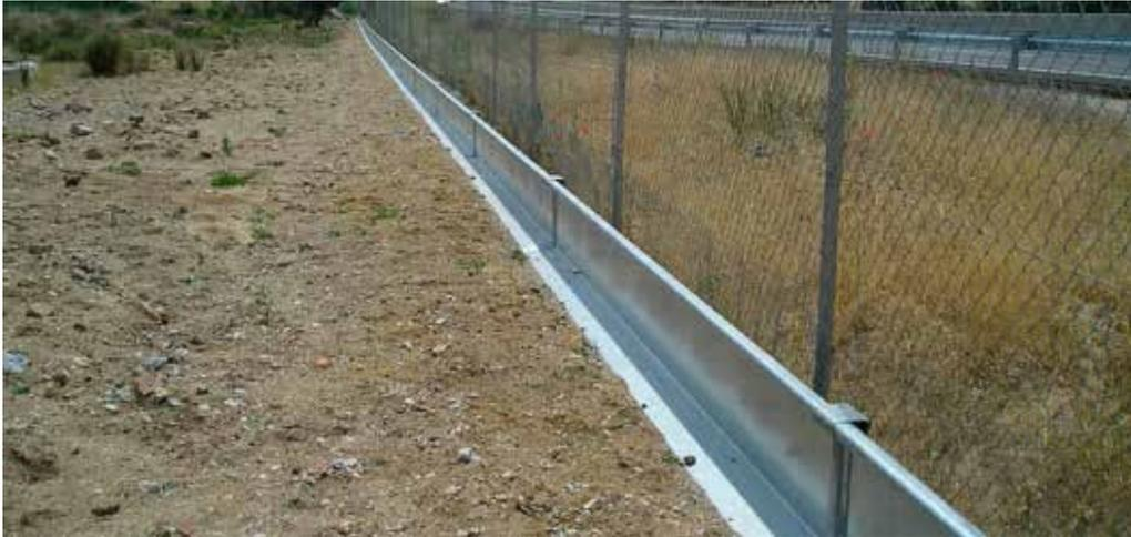
Figure 11.6. Opaque metal structure applied to a fence to guide amphibians towards the crossings. Photo: CEDEX.
