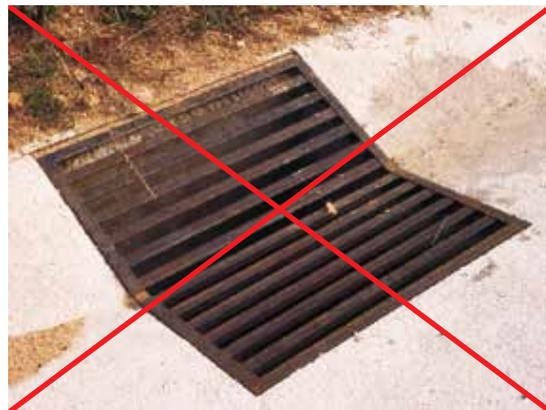
Figure 20.5. Manhole and drain gratings must be dense to prevent small animals from falling inside. The walls of these structures should also be adapted to help animals to escape. Photo: C. Rosell.
