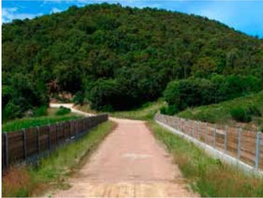
Figure 3.3. Overpass with track in the centre of the structure and two revegetated lateral strips to encourage its use by wildlife. Photo: Territory and Sustainability Department, Government of Catalonia.
