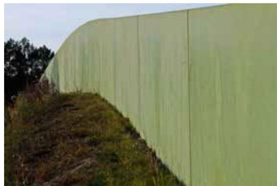
Figure 1.7. Treated timber or stained concrete fences require less maintenance than vegetation. Photo: C. Rosell.
