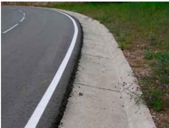
Figure 20.2. Kerb with easy access to the natural environment for animals after crossing a road. Photo: F. Navàs.
