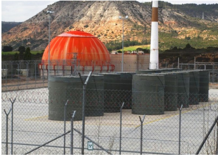
Figure 5. View of the José Cabrera Nuclear Power Plant ITS facility.
