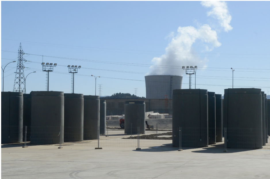
View of the Ascó Nuclear Power Plant ITS.
