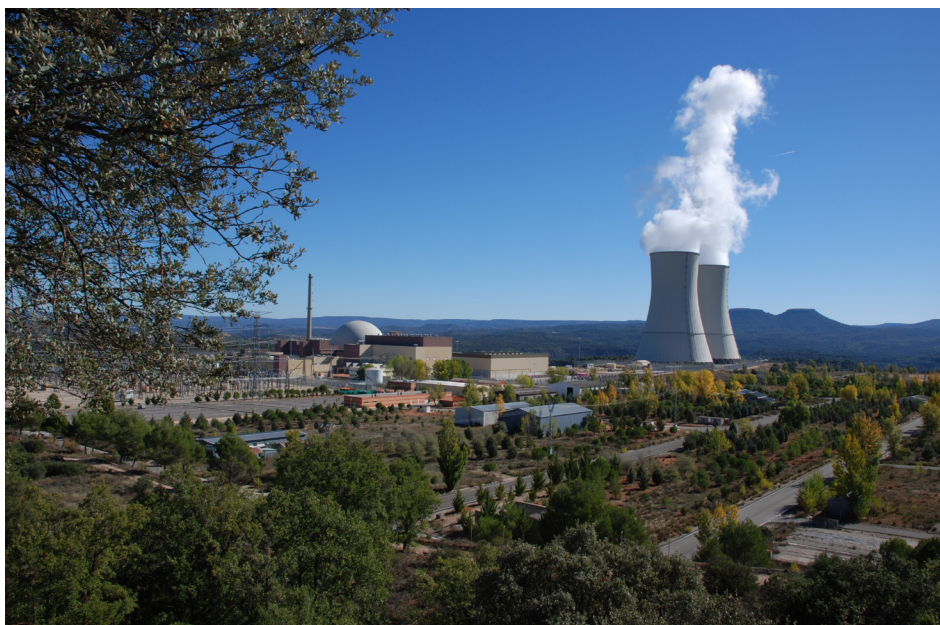
Overview of the Trillo Nuclear Power Plant.
