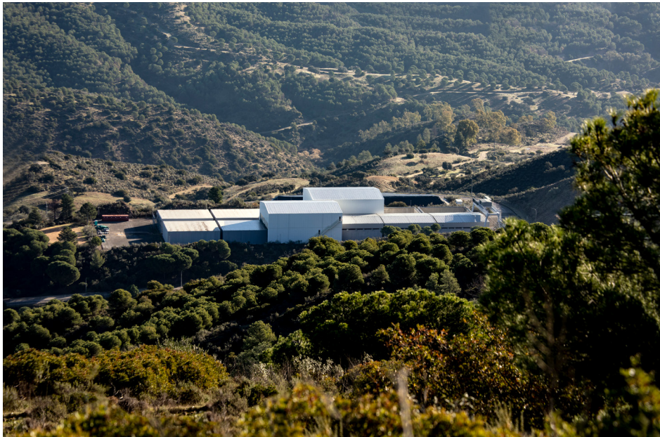
View of the LILW disposal vaults of the Southern Platform of the El Cabril Disposal Facility.
