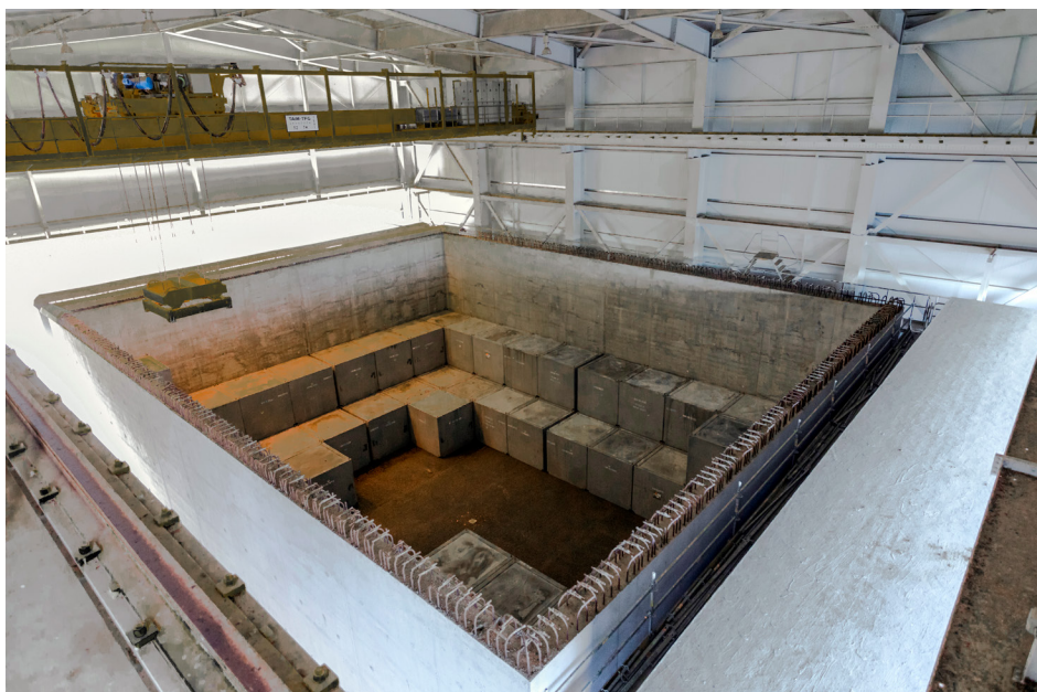
Image of the filling of a LILW disposal vault.
