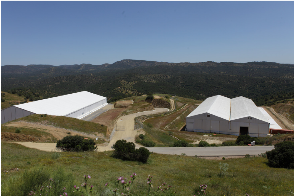
Image of the VLLW disposal vaults at the El Cabril Disposal Facility.
