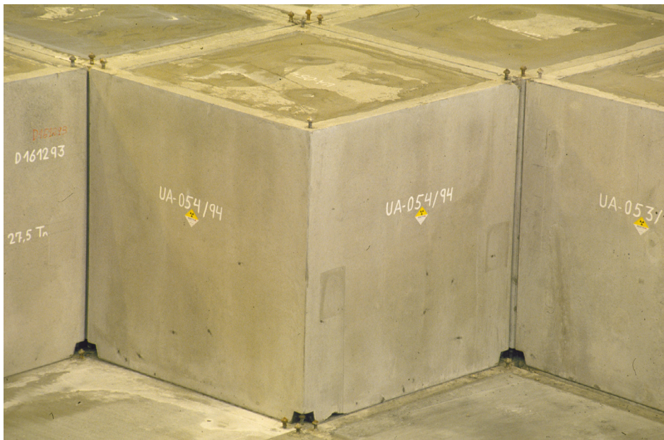
Detail of casks for the disposal of LILW in the disposal vaults of El Cabril.
