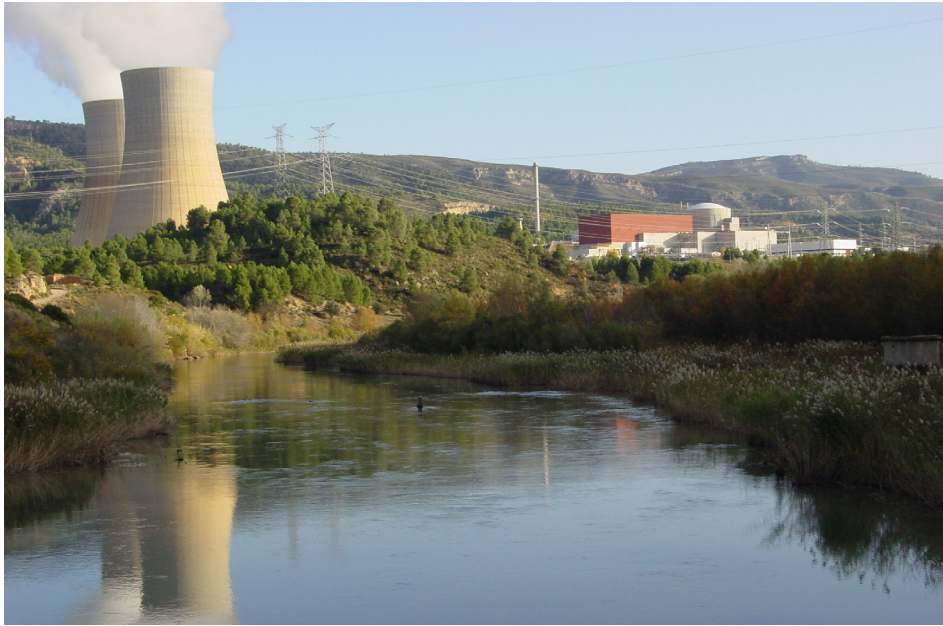
View of the Cofrentes Nuclear Power Plant, Valencia.
