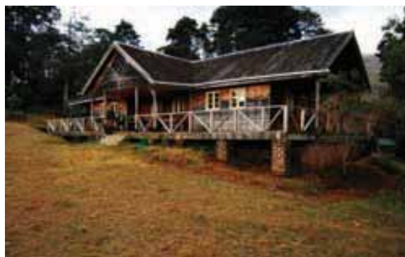
Figure 5: Mountain cottage constructed from Mulanje Cedar timber
