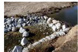
Example of improvement of watercourse morphology. Sediment trap.
