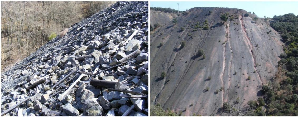
**Figure 34.** Heaps from coal mining extraction showing different durability and fine elements content.
