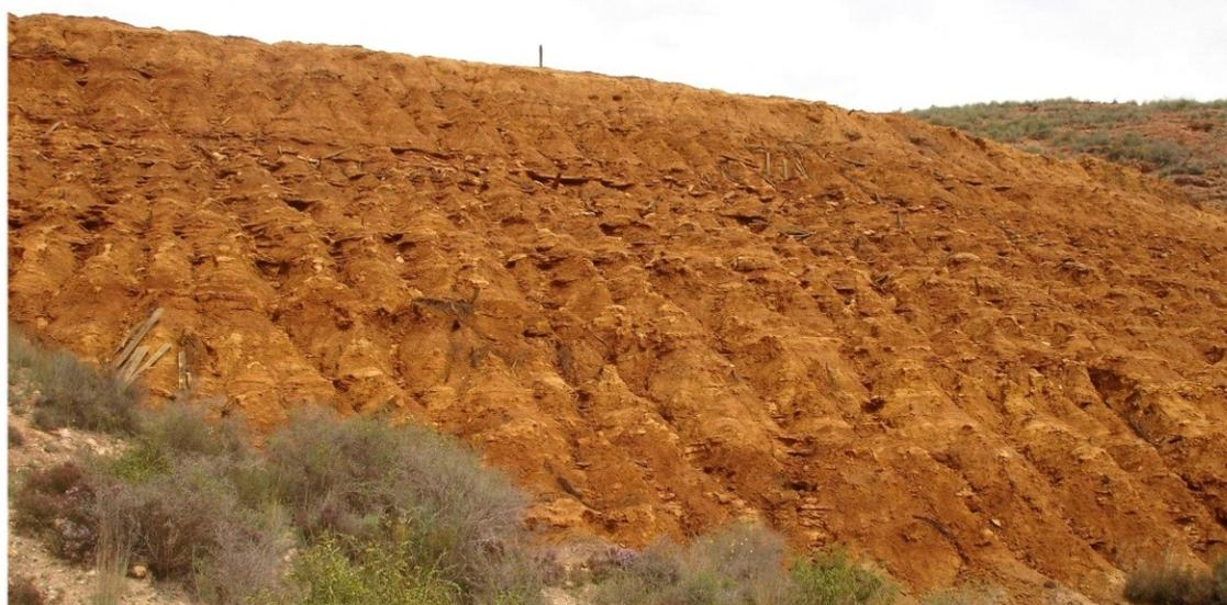
**Figure 28.** Erosion evidences in embankments of mining tailing impoundments. Upper: El Soldado Mine, Villanueva del Duque, Córdoba, Spain. Bottom: Cerro de San Cristóbal, Mazarrón, Murcia, Spain.
