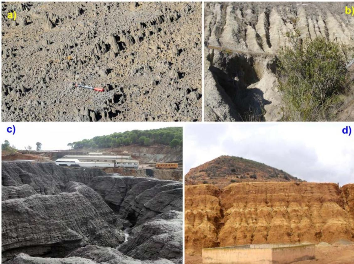
**Figure 42.** Water erosion evidences in embankments of mining tailing impoundments: a) splashing erosion; b) laminar erosion and tubification at the embankment's base; c) gully erosion; d) laminar and gully erosion.
