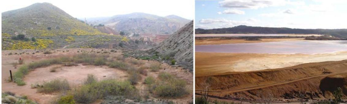
**Figure 44.** Criteria for the identification and delimitation of the settling pond in mining tailing impoundments. Left: settling pond in El Gorguel mining tailing impoundment (Sierra Minera de Cartagena-La Unión, Murcia, Spain), with presence of supernatant, hydrophytic vegetation and precipitated salts. Right: settling pond with supernatant in a mining tailing impoundment in Rio Tinto (Huelva, Spain).
