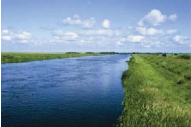
The channelised lower reach of Skjern River.
