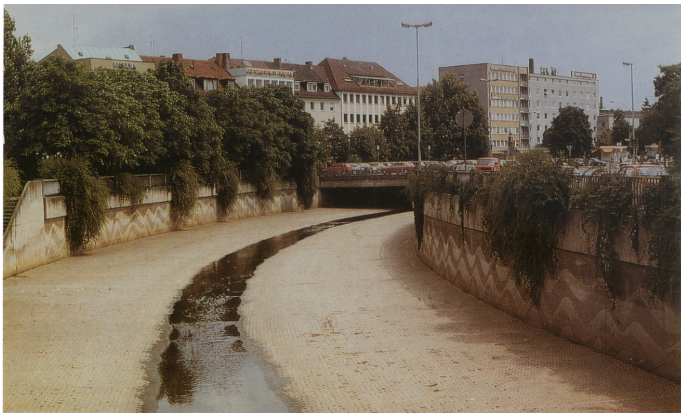
Figure 1. Example of a channelized urban river - a rehabilitation is nearly impossible due to settlements and infrastructure
