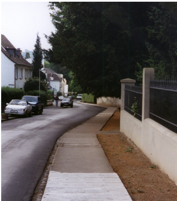
Figure 3. Tubed reach of a small river - the water is located under the flagstones
