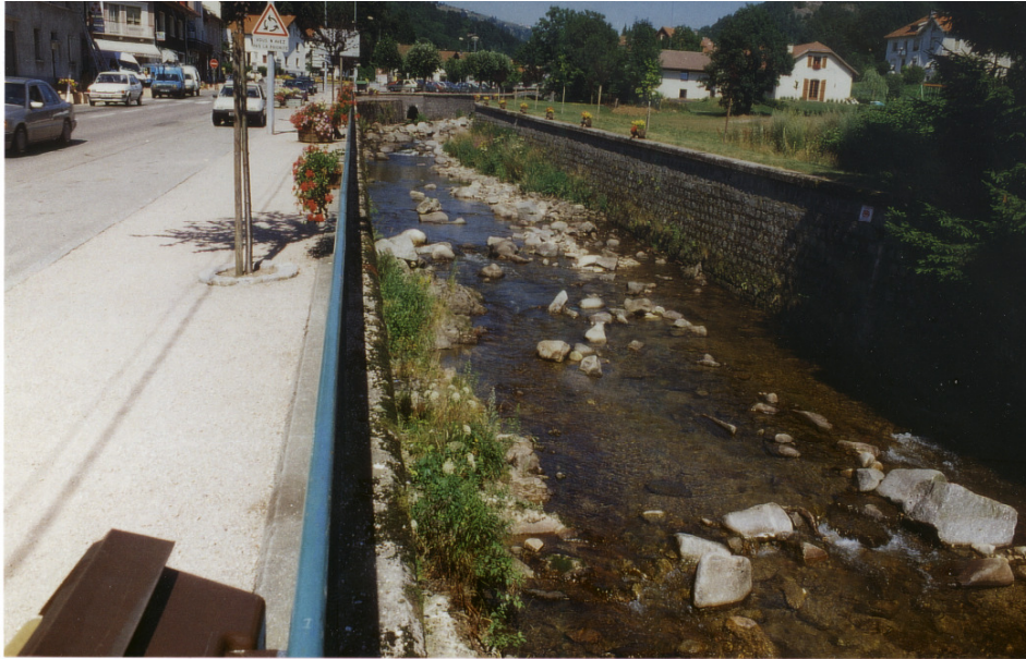
Figure 2. Natural development of an urban river through forming a natural river bottom and typical vegetational cover
