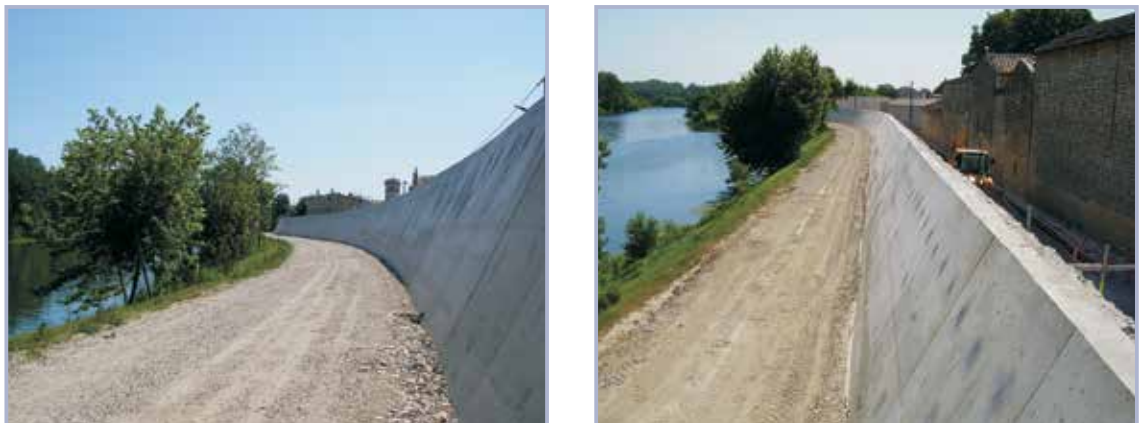
Figure 3.83 Levee crest raising with concrete wall (courtesy T Mallet)
