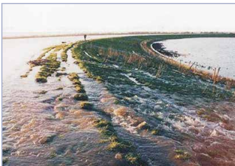
Figure 9.1 Localised overtopping (courtesy Defra)
