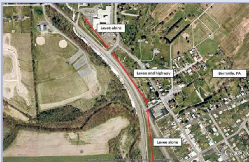
Figure 3.16 Highway embankment serving as line of defence, Bernville, Pennsylvania, USA (courtesy USACE)
