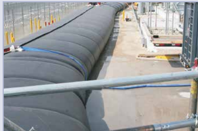
Figure 6.50 Water inflated barrier field setup (courtesy USACE)
