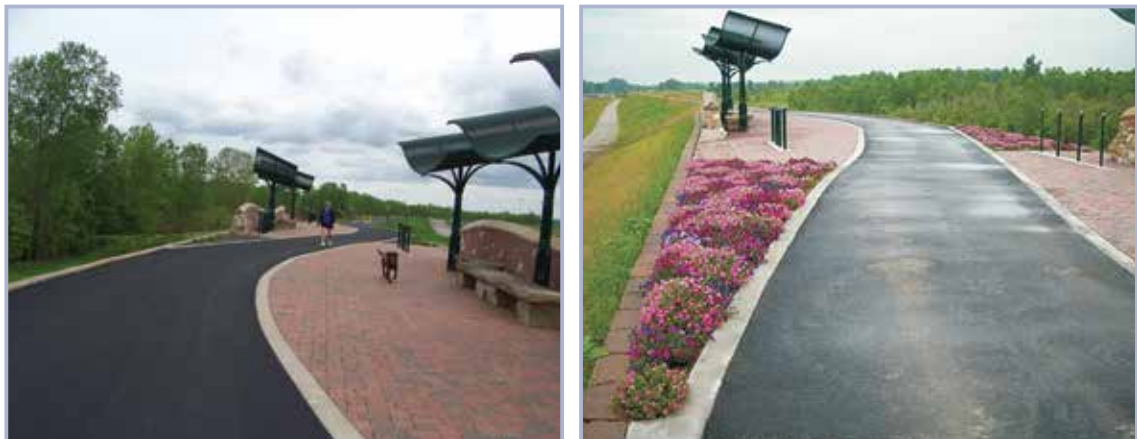
Figure 3.20 Paved/landscaped trails on levee crown, Chesterfield, Missouri, USA
