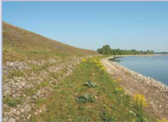
Figure 3.94 Loire levee, Sandillon (courtesy DREAL Centre)
