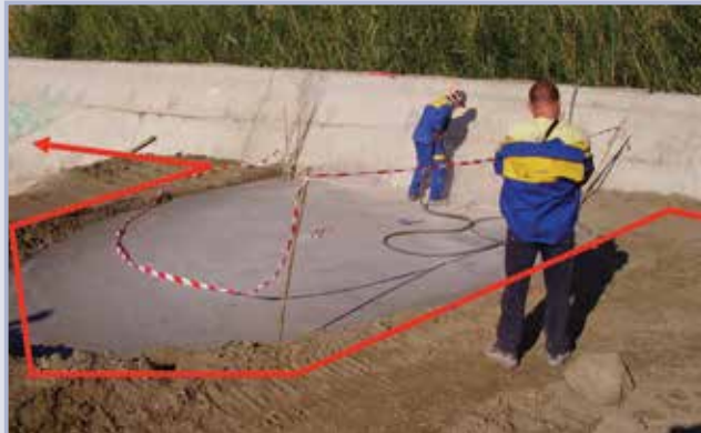
Figure 9.69 Concrete plug installed to lengthen potential seepage path (courtesy Thibaut Mallet)
