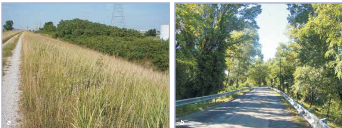
Figure 4.17 Examples of limited visibility and access on levees due to untrimmed grasses and woody vegetation in East St Louis Levee, Illinois, USA (courtesy L F Harder) (a), and France (courtesy M Vennetier) (b)
