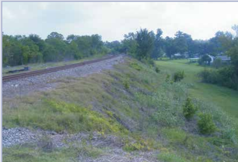
Figure 3.18 Railroad embankment serving as line of defence (courtesy USACE)
