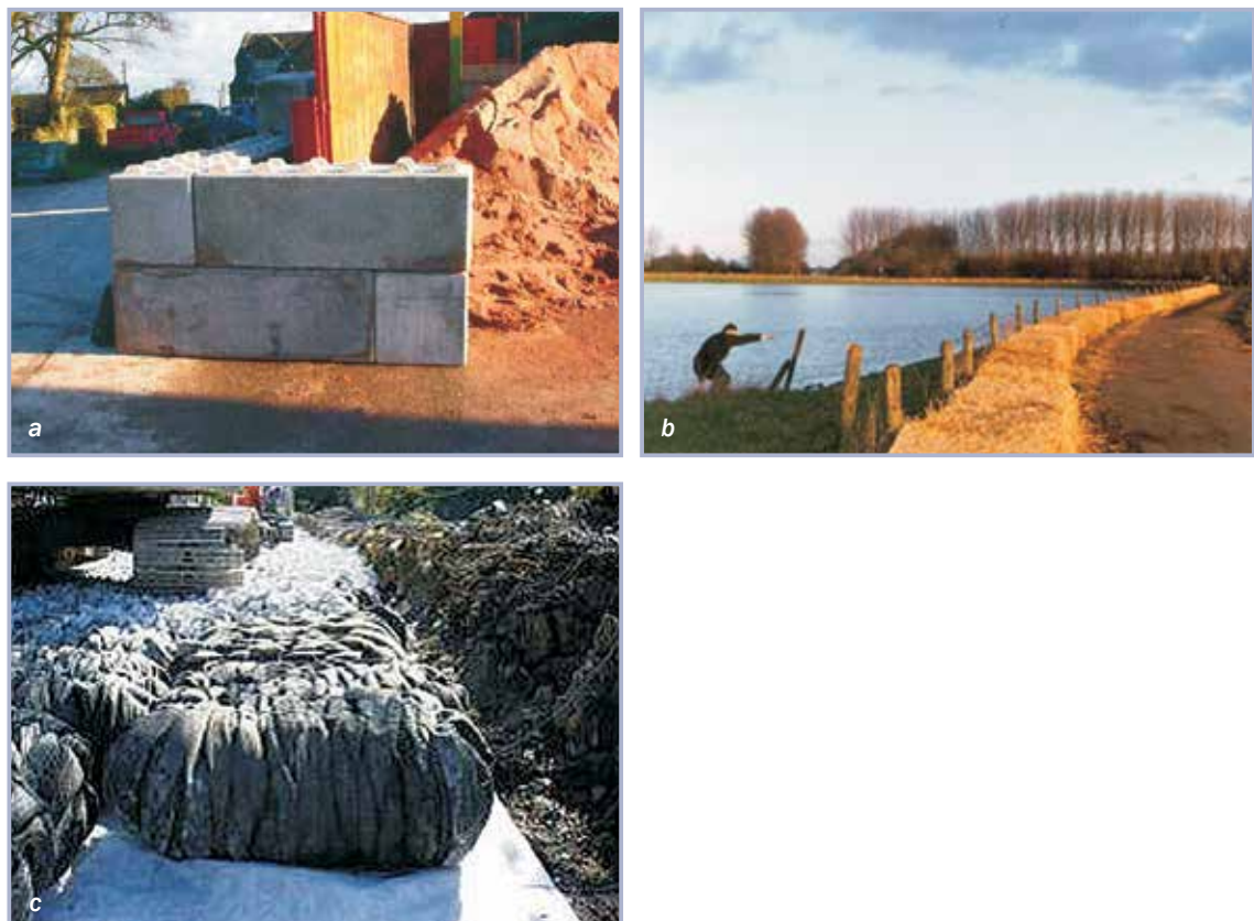
Figure 6.24 Lightweight concrete block (a), straw bales (b), and tyre bales (c) (courtesy Environment Agency)
