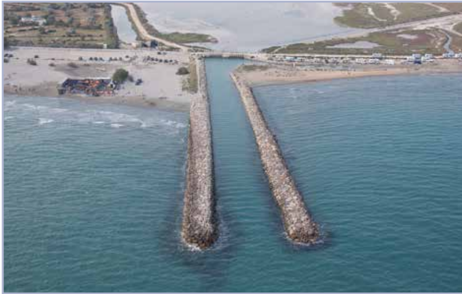
Figure 3.134 Local effect of a groyne (courtesy Symadrem)
