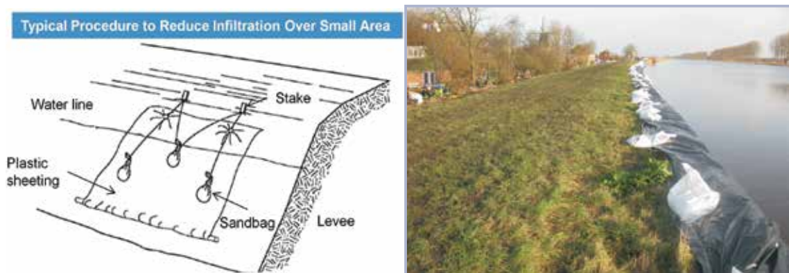
Figure 6.36 Use of impermeable sheeting to reduce infiltration (from DWR, 2010, and courtesy Henk van Hemert)
