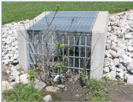
Figure 3.137 Trash screen on upstream pipe end (courtesy USACE)
