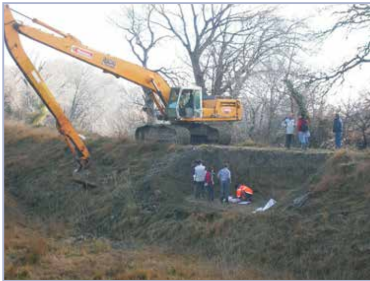
Figure 5.52 Destructive investigation, Rhone River, France (courtesy R Tourment, Irstea)
