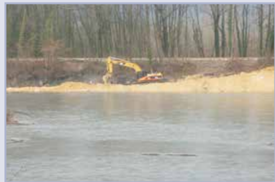
Figure 10.37 The excavator (working on the berm) uses the material to define the profile
