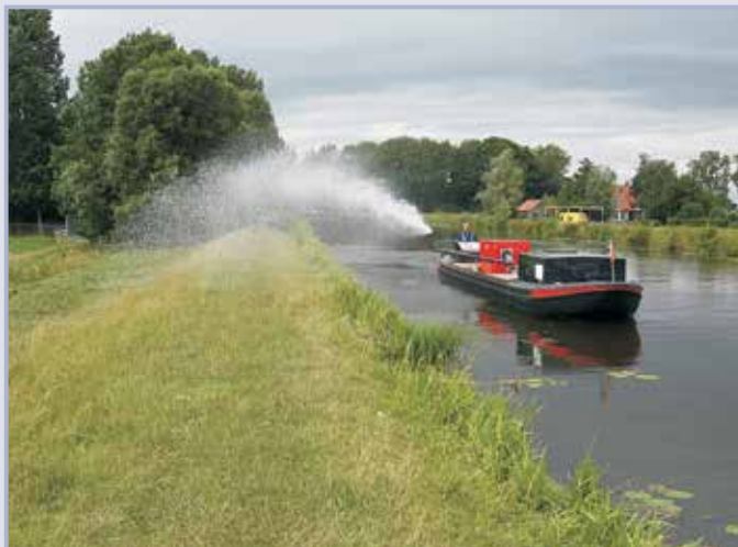
Figure 4.45 Spraying water on levee (courtesy Water Board of De Stichtse Rijnlanden)
