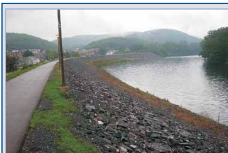
Figure 10.6 Lock Haven Pennsylvania Levee (courtesy Bucharth Horn, Inc)
