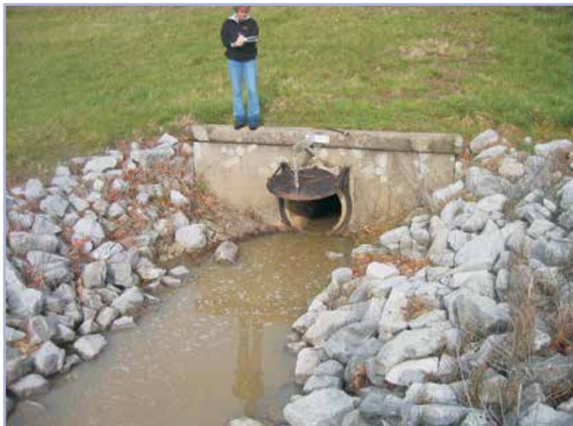
Figure 5.41 Inspection of a culvert outlet (courtesy USACE Louisville District)
