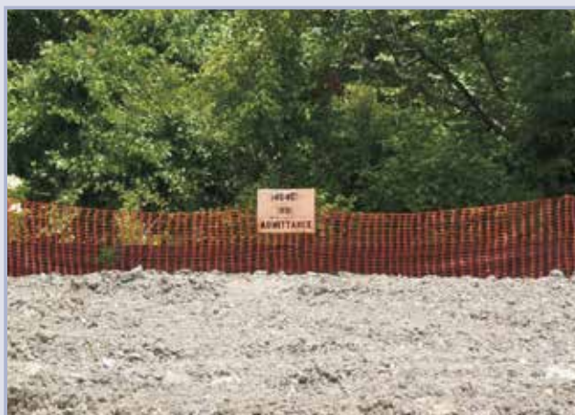
Figure 10.12 Net fencing of a sensitive area (courtesy David St. Marie)
