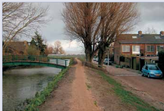
Figure 4.26 Trees on the landside slope of the regional (secondary) levee along the canal Pijnackerse (courtesy STOWA)
