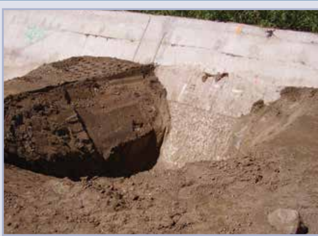
Figure 9.68 Excavation of trench perpendicular to seepage path (courtesy Thibaut Mallet)
