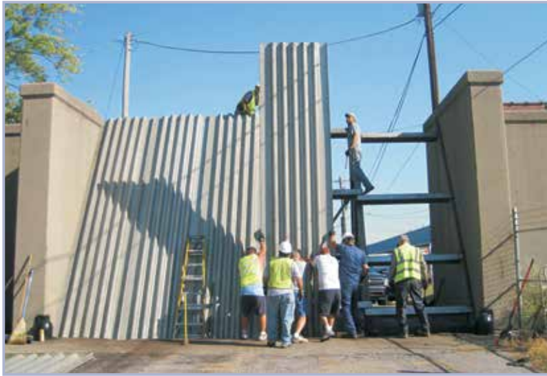
Figure 5.42 Inspection during a closure installation (courtesy USACE Louisville District)
