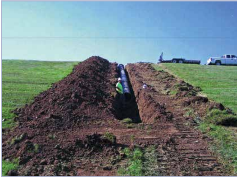
Figure 3.142 Utility line installation (courtesy Lawrenceburg Indiana Levee System, Louisville District, USACE)
