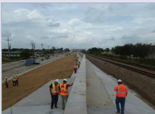
Figure 9.147 Portion of LPV 105 constructed T-wall (courtesy Barry Fehl/URS)
