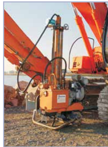
CPT rams on long reach excavator (courtesy Fugro)
