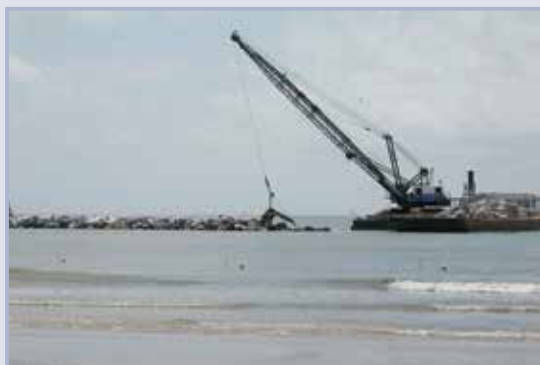
Figure 10.43 Repairs to breakwaters along Grand Isle, LA, USA (courtesy USACE)
