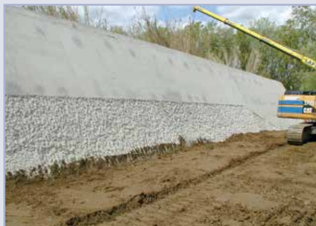
Figure 9.66 Preparation of the flood wall transition at Comps (courtesy Thibaut Mallet)
