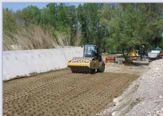
Figure 9.67 Compaction of levee fill against flood wall transition (courtesy Thibaut Mallet)
