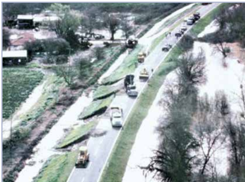
Figure 9.51 Slope stability failure due to elevated pore pressures during high water in the Sacramento River on the Natomas Levee in California, USA (courtesy Mary Perlea, USACE)
