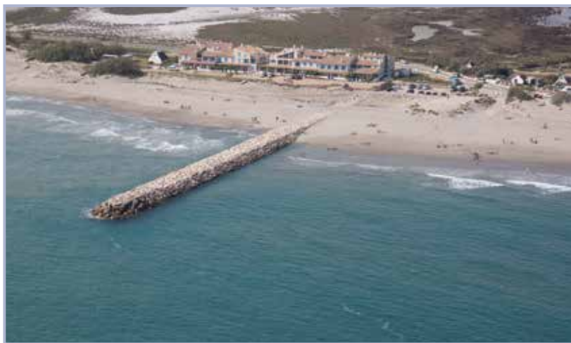
Figure 3.133 Groynes – large-scale view (courtesy Symadrem)
