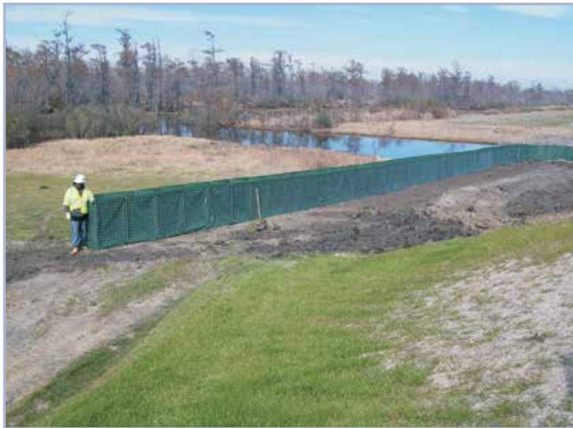
Figure 10.8 Example of temporary flood protection during construction (courtesy USACE)
