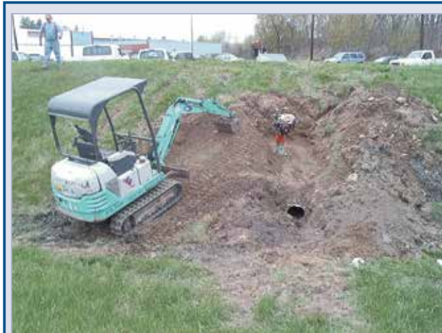
Figure 4.7 Unauthorised pipe installed by local business had to be abandoned and sealed at its expense
