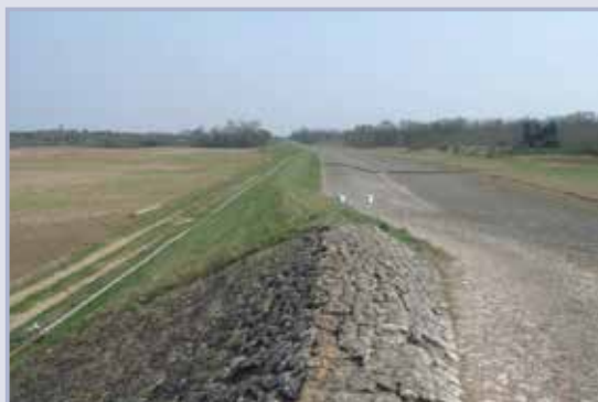
Figure 9.131 Jargeau weir with its 715 m long, 1.5 m high, grassy bench fuse (Degoutte et al, 2012)
