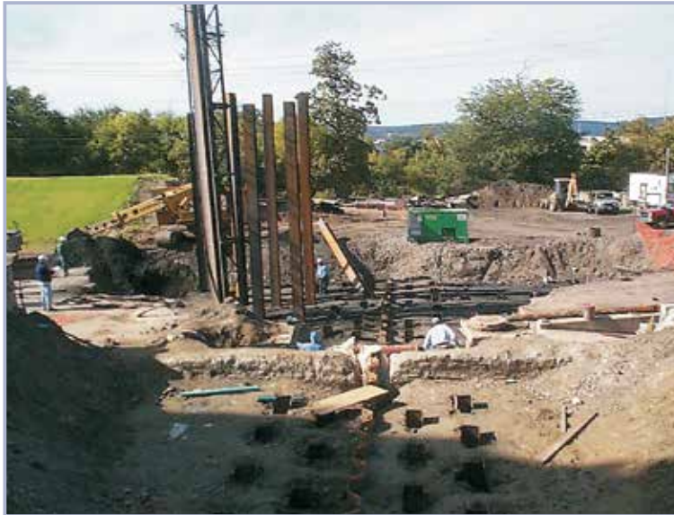
Figure 10.67 H-pile foundation for a closure structure foundation (courtesy USACE)
