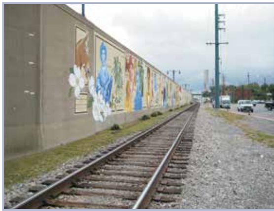
Figure 3.102 Painted concrete flood wall improvements, Cape Girardeau, Missouri, USA (courtesy USACE)
