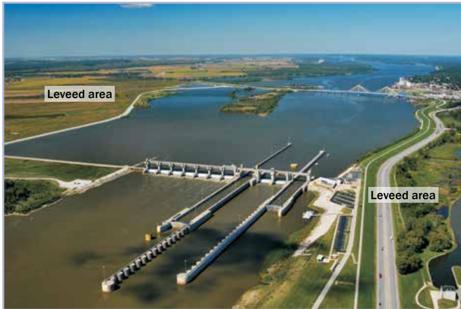
Figure 3.10 Mississippi river lock and dam (adapted by Y Deniaud)
