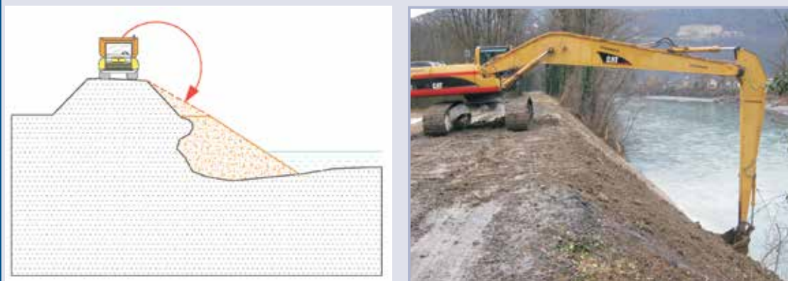
Figure 10.40 Excavator working from crest
