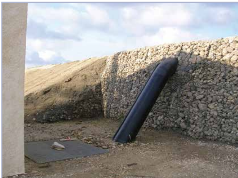
Figure 9.155 Landward side of pipe crossing of Rhône river in France (courtesy Symadrem)
