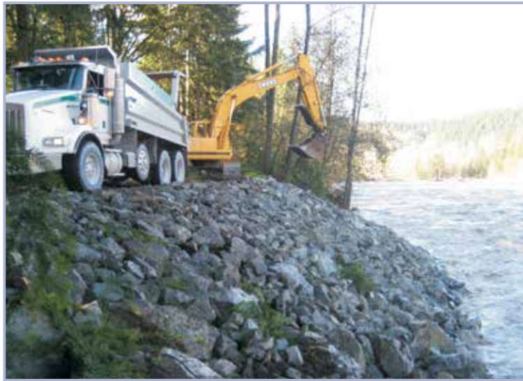
Figure 6.28 Construction of a rock revetment (courtesy USACE)
