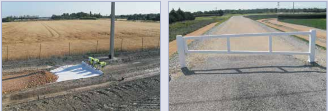
Figure 10.33 Access road and security gate (courtesy EGIS)
