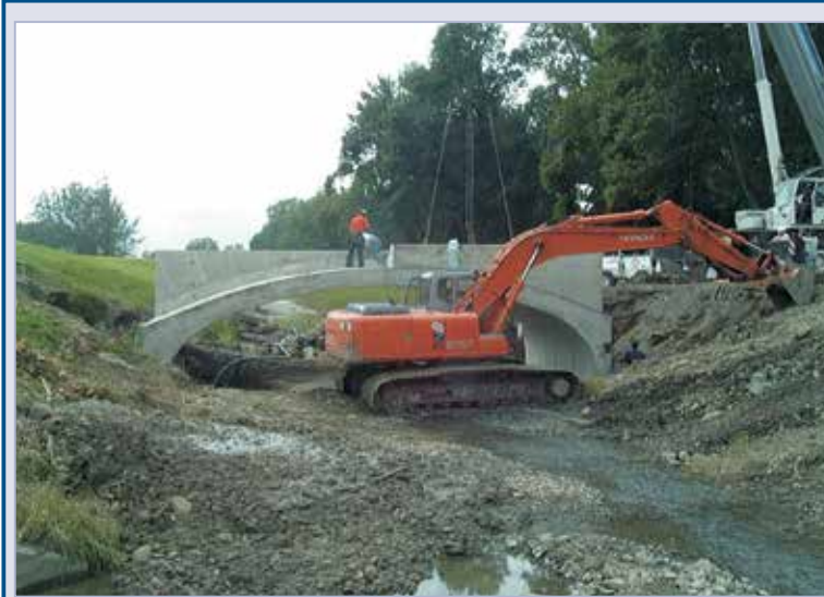
Figure 4.15 Permitted bridge installation in Riverside, New York, USA
