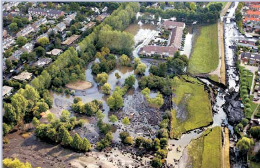
Figure 3.160 Translational sliding in Wilnis Levee (courtesy STOWA)
