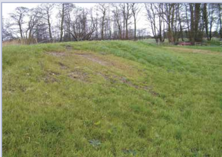
Figure 9.85 Levee constructed of peat and gravel, Broadlands, UK (courtesy BAM Nuttall, and CH2MHill)
