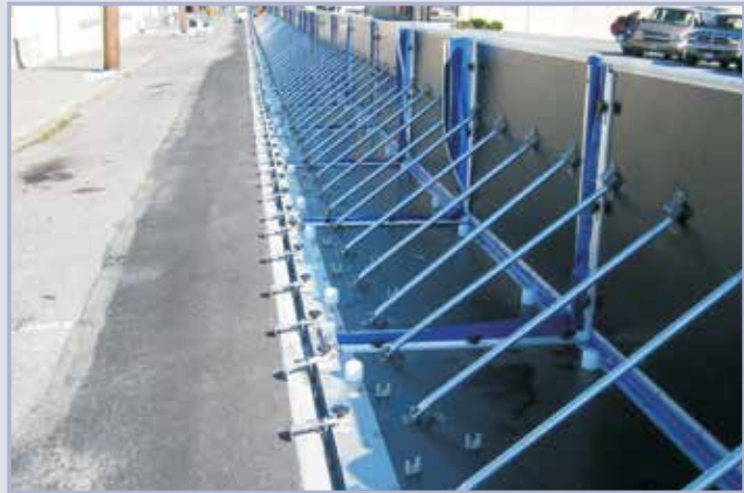
Figure 6.49 AquaFence implementation (courtesy USACE)
