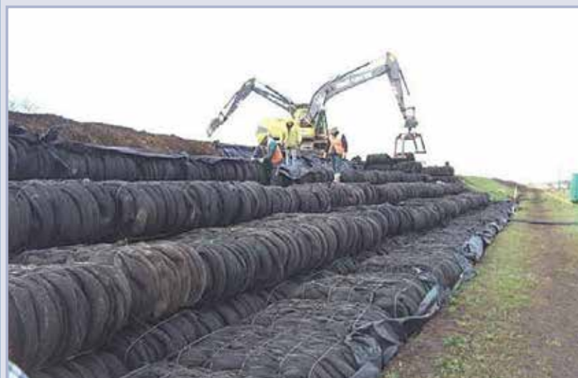
Figure 9.108 Tyre bale placement completed on one levee segment (courtesy Environment Agency)
