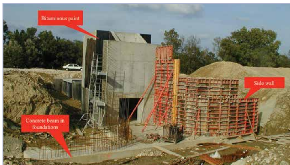
Figure 9.164 Construction of hydraulic structures crossing at Aramon (courtesy Thibaut Mallet)
