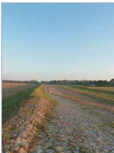
Figure 3.98 Spillway on the Loire River (courtesy Y Deniaud, CETMEF)
