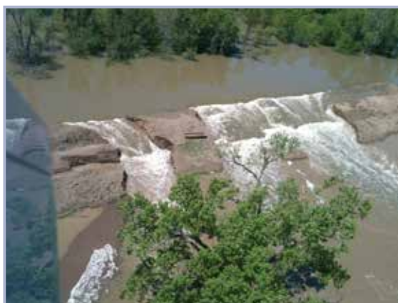
a Overhead view showing overtopping in sacrificial levee section
