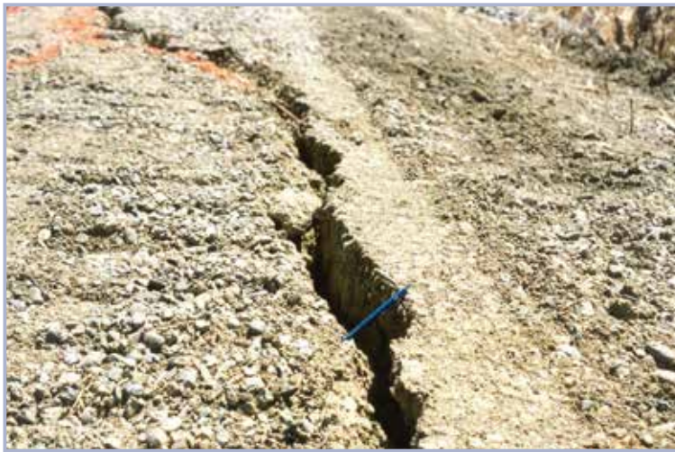
Figure 9.78 Head scarp of a slide on the levee crest (courtesy Said Salah-Mars, URS Oakland)
