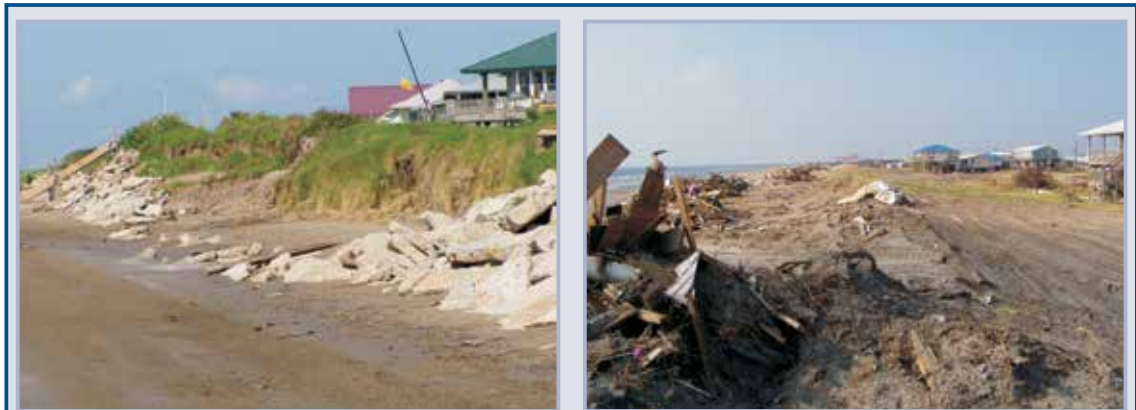
Figure 10.41 Hurricane damages in Grand Isle, LA, USA (courtesy USACE)
