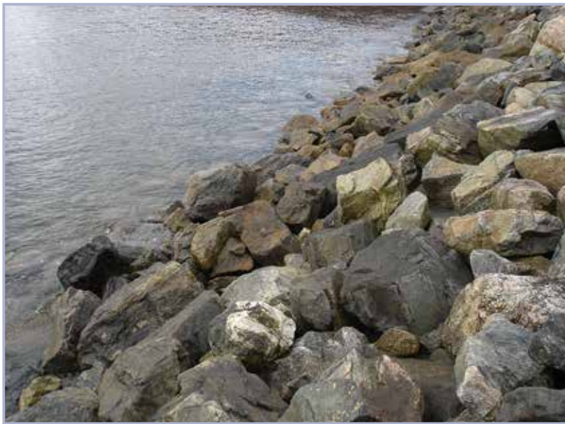
Figure 9.26 Armourstone revetment (courtesy William Allsop, HR Wallingford)
