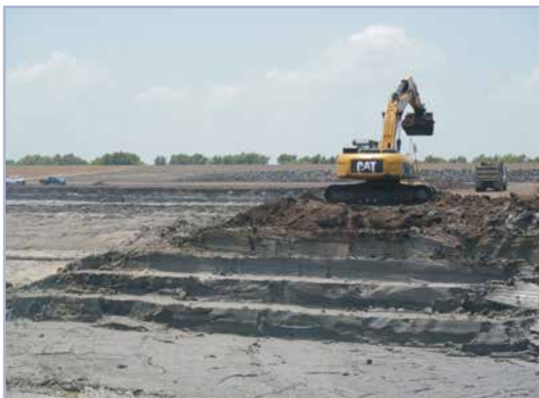
Figure 10.17 Hydraulic excavator handling soil (courtesy USACE)
