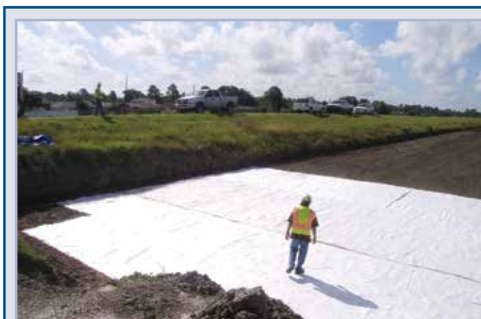
Figure 9.105 High strength geotextile used at the base of the New Orleans levee (courtesy Mike Wielputz, USACE)
