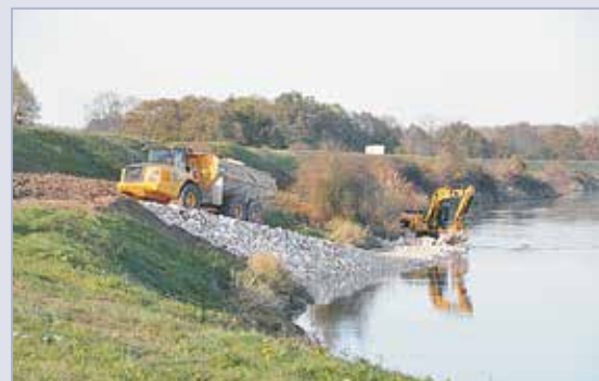
Figure 4.53 Placing rip-rap at levee toe (courtesy DREAL Centre)
