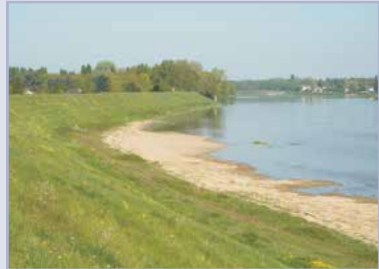
Figure 3.95 Loire levee, Melleray (courtesy DREAL Centre)
