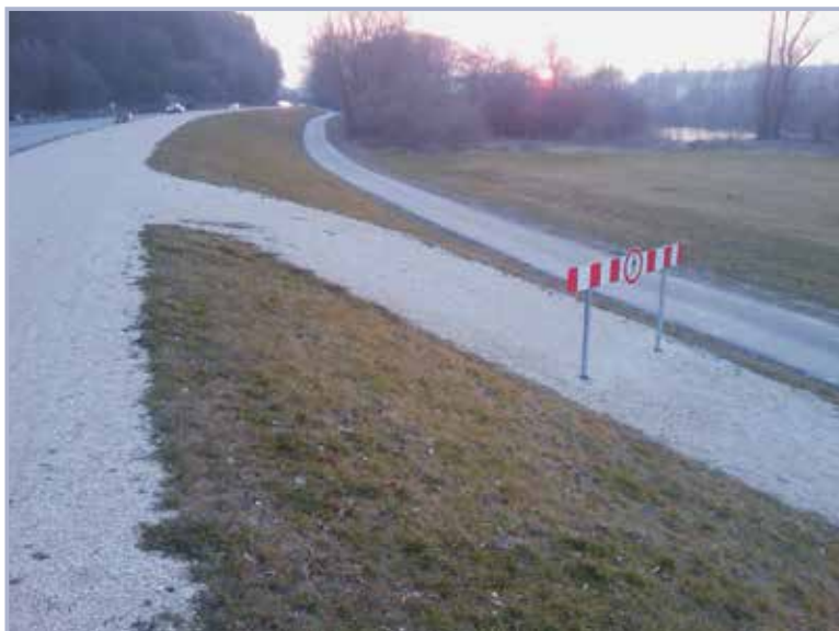
Figure 3.15 Danube levee access ramp near Regensburg, Germany (courtesy Reinhard Pohl)
