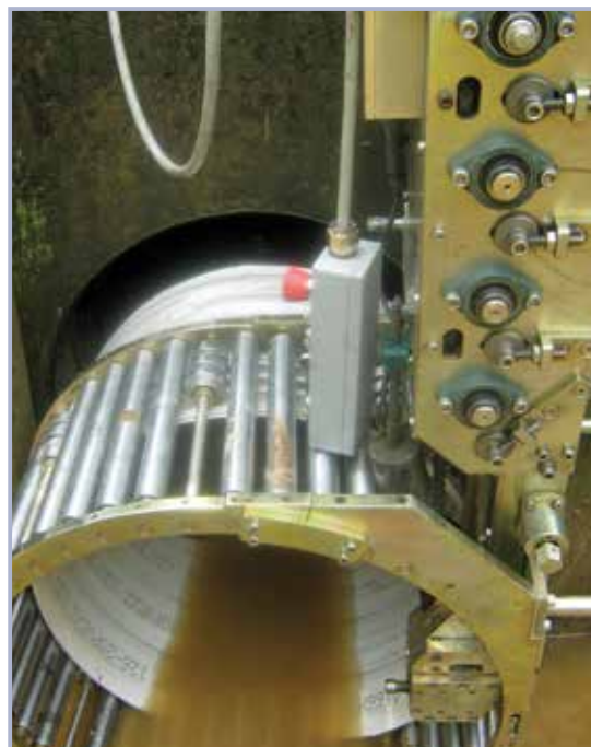
Figure 10.73 Typical installation of a spiral wound pipe liner, Jeffersonville/Clarksville Levee System in Indiana, USA (courtesy Christina Neutz)
