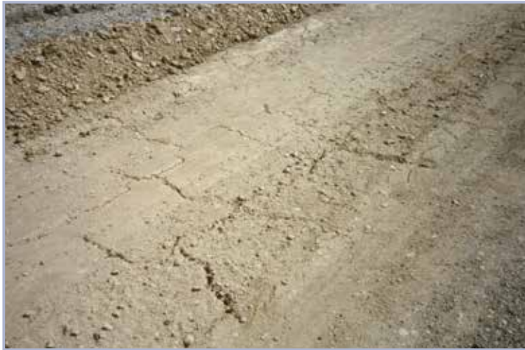
Figure 9.77 Formation of 'alligator skin' type appearance (courtesy Said Salah-Mars, URS Oakland)
