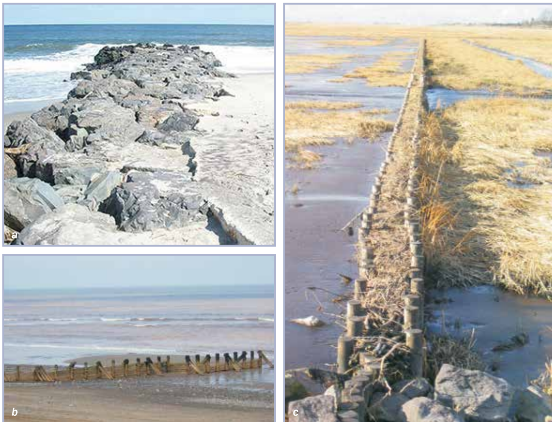
Figure 6.30 Examples of rock groyne (a), timber groyne (b), and earthfill groyne (c) (courtesy Wikimedia Commons)
