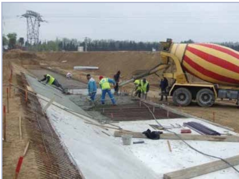
Figure 9.118 Construction of reinforced concrete spillway slabs (after Degoutte et al, 2012)
