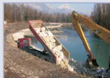
Figure 10.61 Truck uses berm to supply excavator with rip-rap for placement
