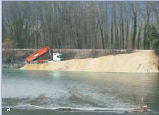
Figure 10.36 Truck dumping armourstone (a), and loader placing armourstone (b)
