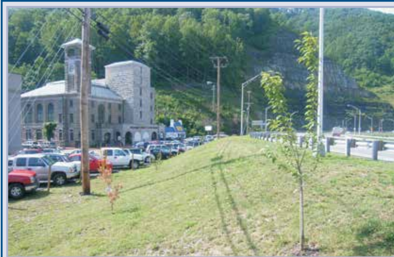
Figure 3.17 Highway embankment serving as line of defence (courtesy USACE)
