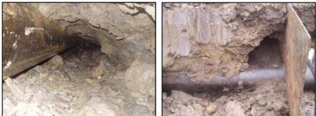
Figure 9.157 Internal erosion around pipes caused by poor compaction and hydraulic separation (from FEMA, 2009, courtesy FEMA and US Bureau of Reclamation)
