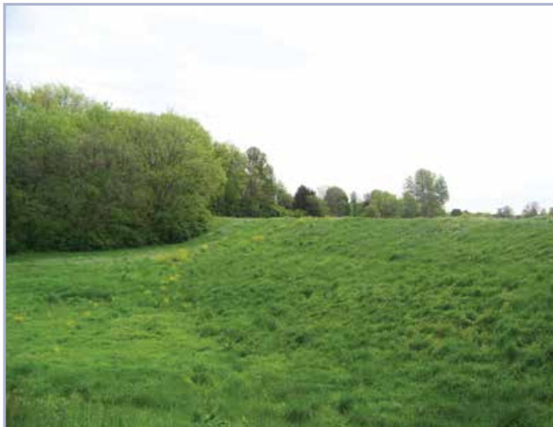
Figure 3.150 Transition in terms of the geometry: transition from levee in to hillside, Columbia, Illinois, USA (courtesy St Louis District, USACE)
