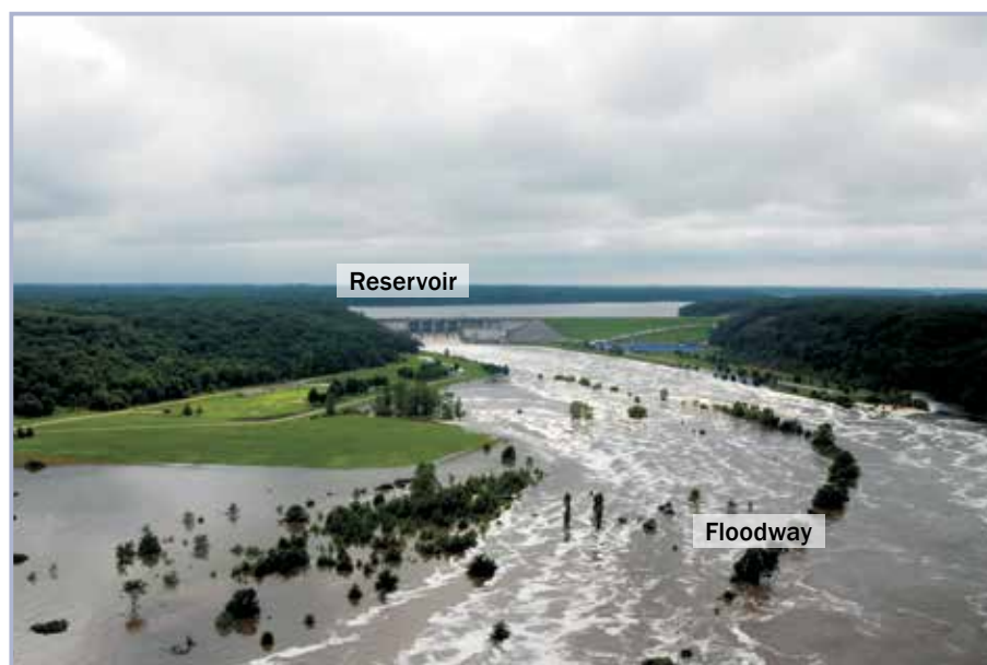
Figure 3.9 Spillway release from a reservoir (adapted by Y Deniaud)
