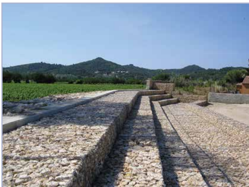
Figure 9.125 Stepped gabion weir downstream of Comps, France (Degoutte et al. , 2012)
