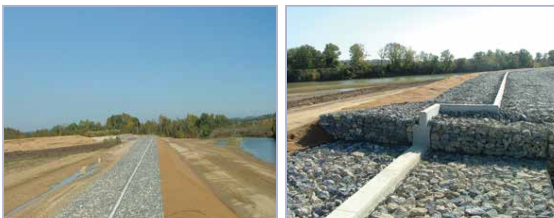
Figure 9.123 Lunel spillway on the Vidourie River, France, (Degoutte et al, 2012)
