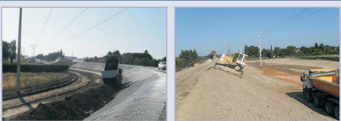
Figure 10.32 Topping of the embankment with topsoil (courtesy EGIS)
