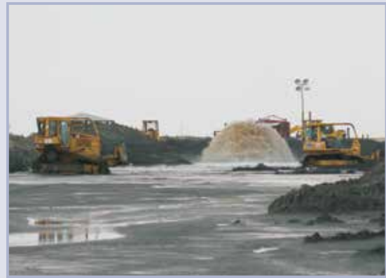
Figure 10.45 Sand placement operations at discharge pipe (courtesy USACE)
