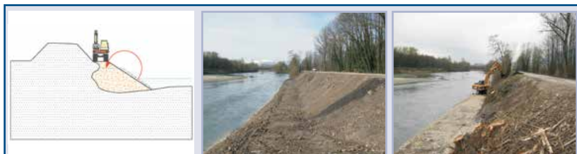
Figure 10.39 Excavator working on berm
