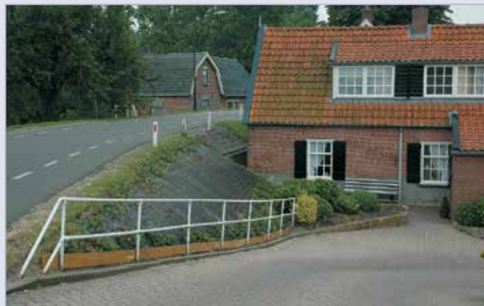
Figure 4.12 Levee along a river – historical house on the riverside of the levee, the Netherlands
