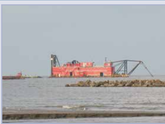
Figure 10.44 Dredging operations at offshore borrow site (courtesy USACE)
