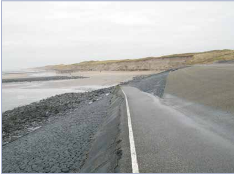
Figure 3.153 Transition erosion dune north of coastal levee Hondsbossche-en Pettemerzeewering, the Netherlands (courtesy H Van Hemert)
