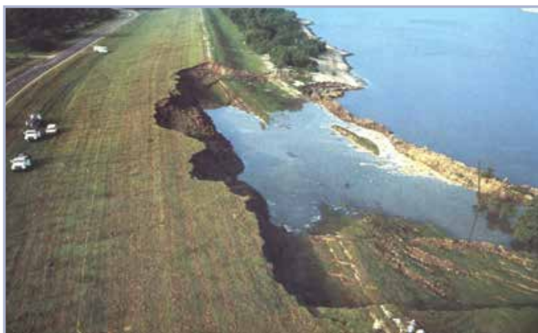
Figure 9.54 Mississippi River failure attributed to rapid draw-down (USACE, 2003)
