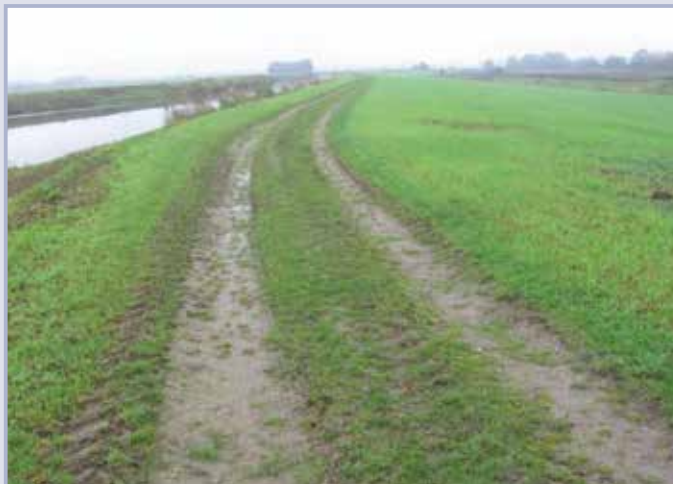
Figure 9.127 Looking downstream along spillway crest (courtesy Black and Veatch Ltd and Environment Agency)
