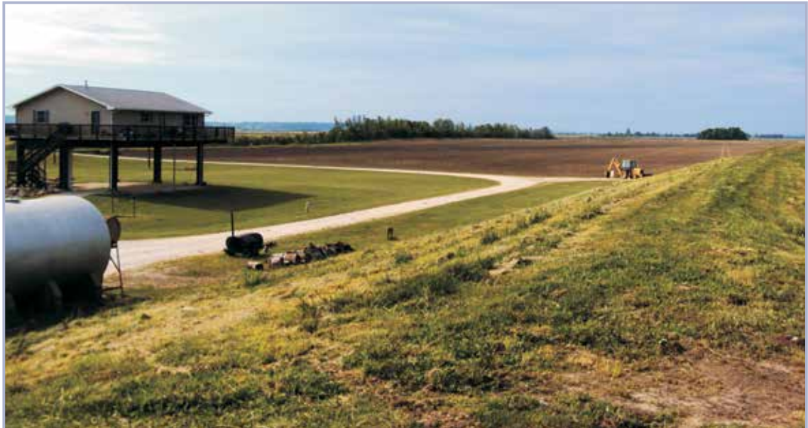
Figure 2.10 Development policy in practice – an elevated construction technique used to reduce the impacts and damage of flooding to a home near the Illinois River, St Louis District, USA (courtesy USACE)
