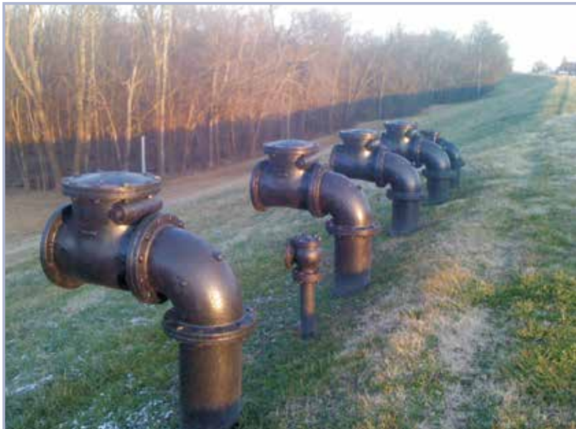
Figure 3.136 Air relief valves on levee crest (courtesy Paducah Kentucky Levee System, Louisville District, USACE)
