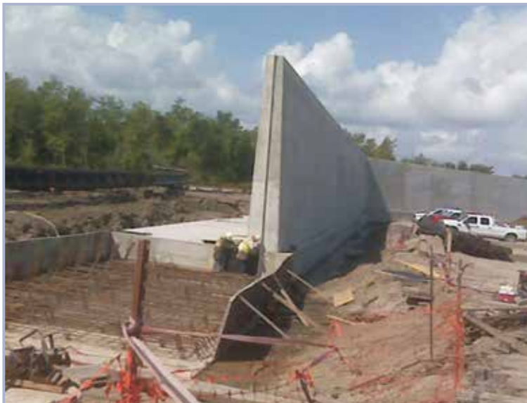
Figure 10.68 Concrete flood wall (courtesy USACE)
