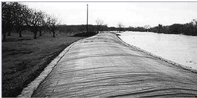
Figure 6.33 Use of emergency spillway (State of California, 2010)
