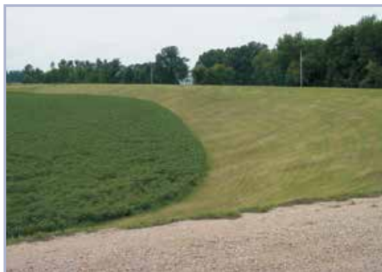
Figure 4.62 Levee tying into high round (Halstad, Minnesota, USA)
