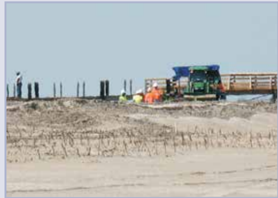
Figure 10.47 Vegetation planting operations (courtesy USACE)
