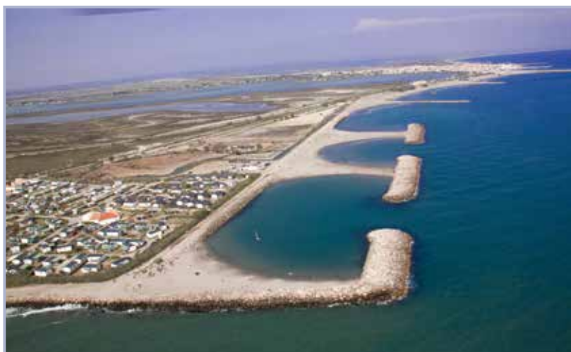
Figure 3.130 Detached breakwaters in Les Saintes-Maries-de-la-Mer, Mediterranean sea, France (courtesy Symadrem)
