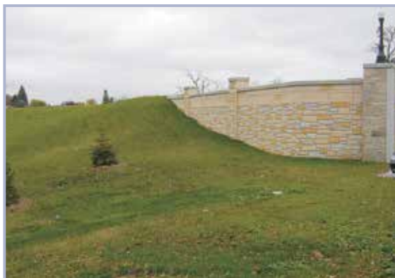
Figure 4.61 Transition from flood wall to levee (Rushford, Minnesota, USA)
