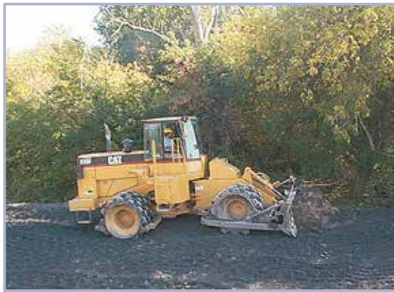
Figure 10.24 Verification of required number of passes of a self-propelled compactor to achieve specified density. This type of machine would count as two passes, since there are compaction drums on both axles (courtesy USACE)
