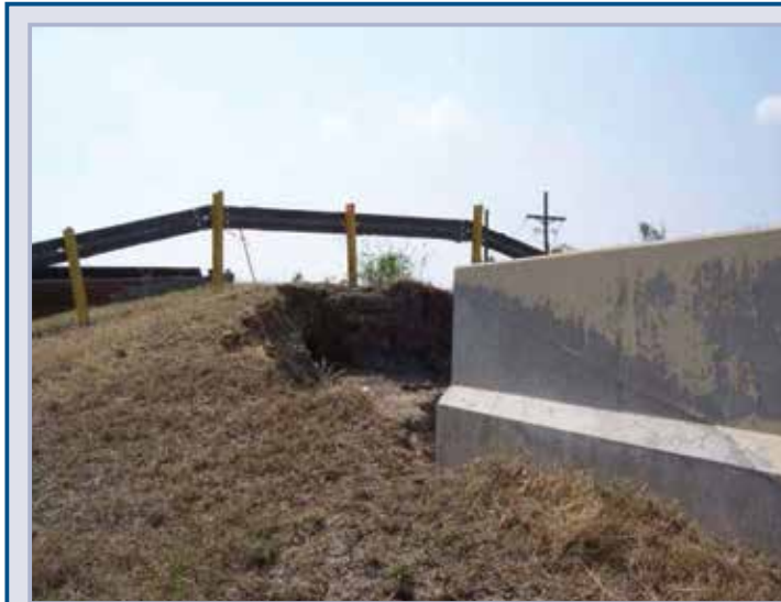
Figure 9.65 New Orleans levee scour at transition with a flood wall (courtesy USACE)
