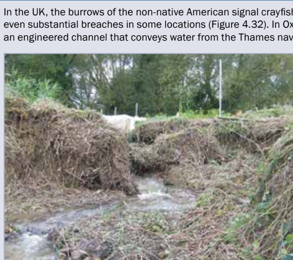
Figure 4.32 Breach in Wolvercote Millstream bank, England, caused by signal crayfish activity (courtesy Environment Agency)
