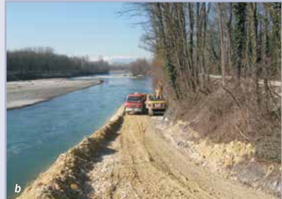
Figure 10.36 Truck dumping armourstone (a), and loader placing armourstone (b)
