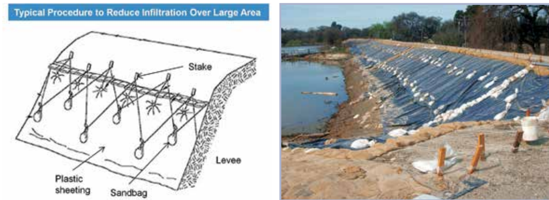
Figure 6.35 Use of impermeable sheeting to reduce infiltration over large area (a) and field application (b) (from DWR, 2010 and courtesy USACE)
