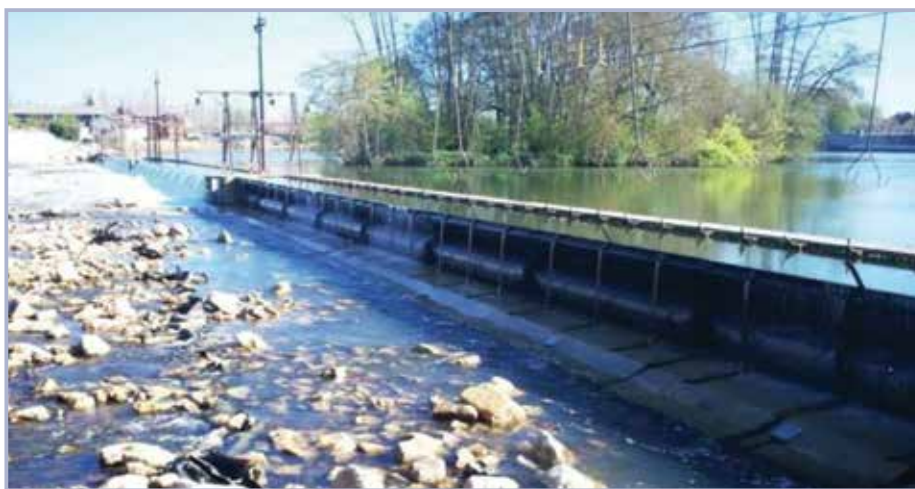
Figure 9.136 Inflatable metal-flap thresholds at Auxonne (Degoutte et al , 2012)
