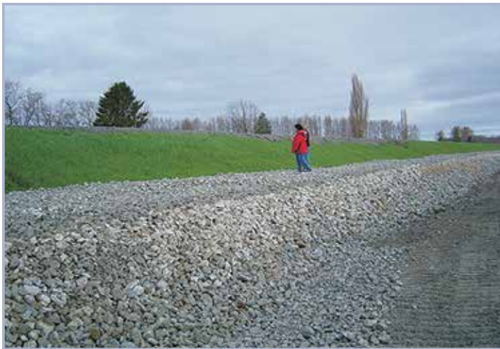
Figure 6.37 Seepage berm constructed landside of levee (courtesy USACE)
