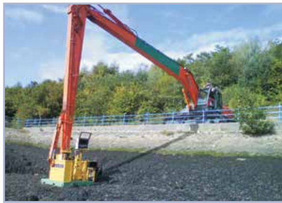
CPT rams on long reach excavator (courtesy Lankelma)
