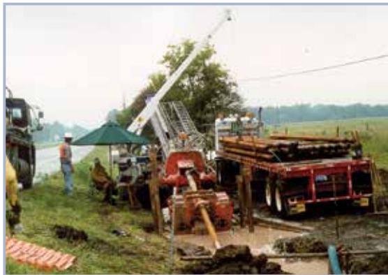
Figure 3.143 Directional drilling operation (courtesy USACE)
