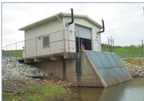
Figure 3.139 Pumping station (courtesy St Louis District, USACE)
