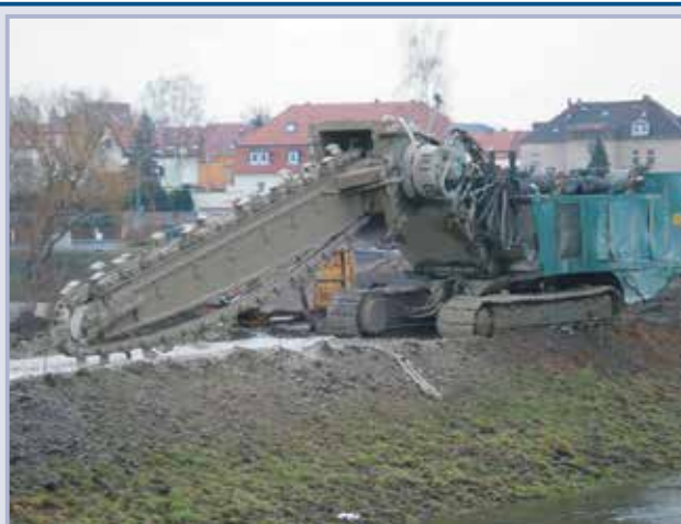
Figure 10.52 Milling-mix technique (FIM) on a levee. The sword of the soil cutting and mixing machine breaks up the soil and feeds in the binder suspension
