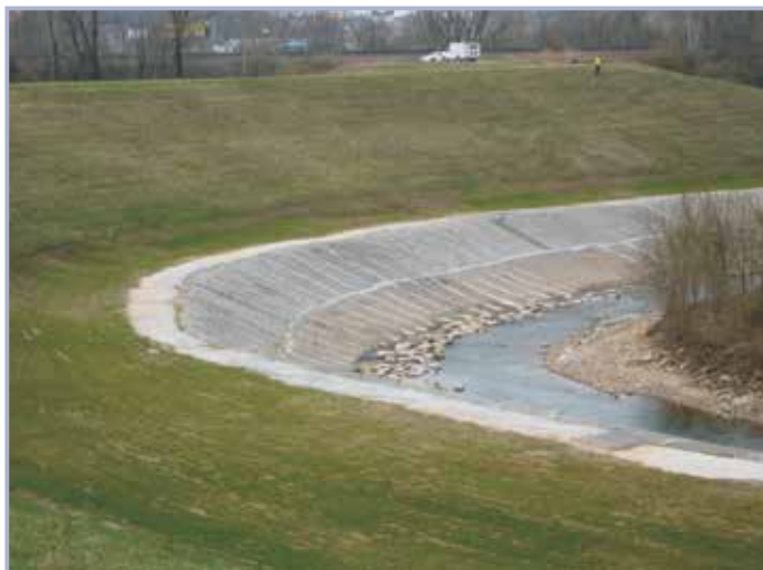
Figure 3.34 Articulated mat along creek channel (courtesy St Louis District, USACE)
