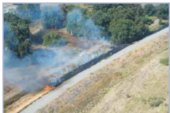
Figure 4.21 Burning of levee slope in California, USA (courtesy L F Harder)
