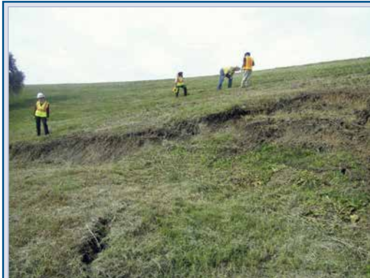
Figure 5.40 Slope movement on the Dallas levee system, Texas, USA (courtesy USACE Fort Worth District)
