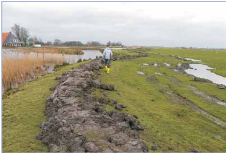
Figure 6.22 Increase crest height with bare soil (clay) (courtesy Wetterskip Fryslân)
