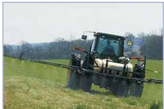
Figure 4.19 Mechanical application of a broadleaf herbicide on a grass levee slope
