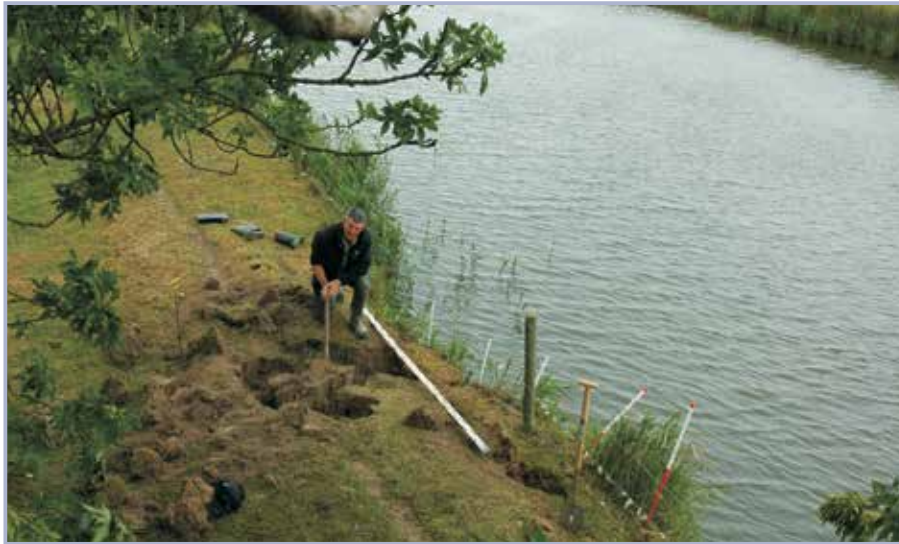
Figure 3.27 Opened burrow of musk rat, levee along canal in Friesland (NL) (courtesy Henk Van Hemert)
