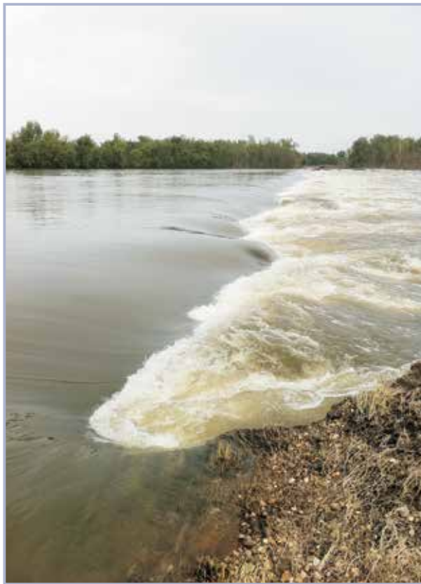
Figure 8.16 Water overflowing a levee with significant energy dissipation where accelerated flow interacts with tailwater the levee crown has been substantially eroded by the overflow (courtesy USACE)
