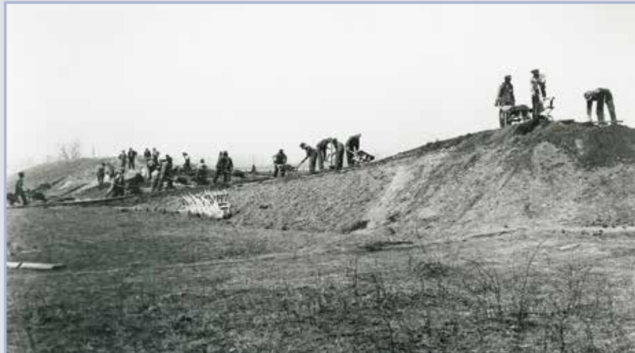
Figure 3.41 Early construction of levees (courtesy USACE)
