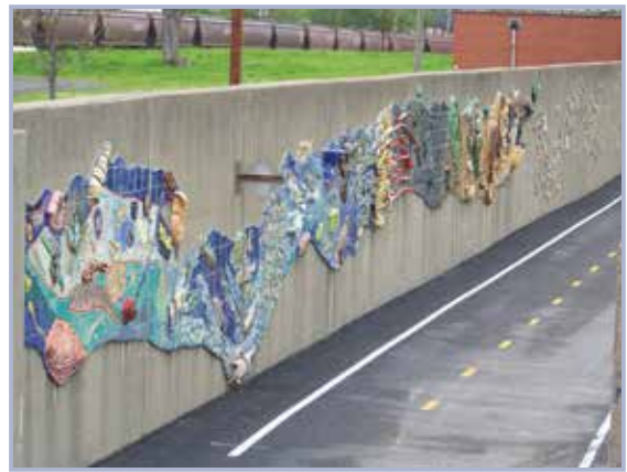
Figure 3.103 Flood wall with aesthetic, St Louis, Missouri, USA (courtesy USACE)
