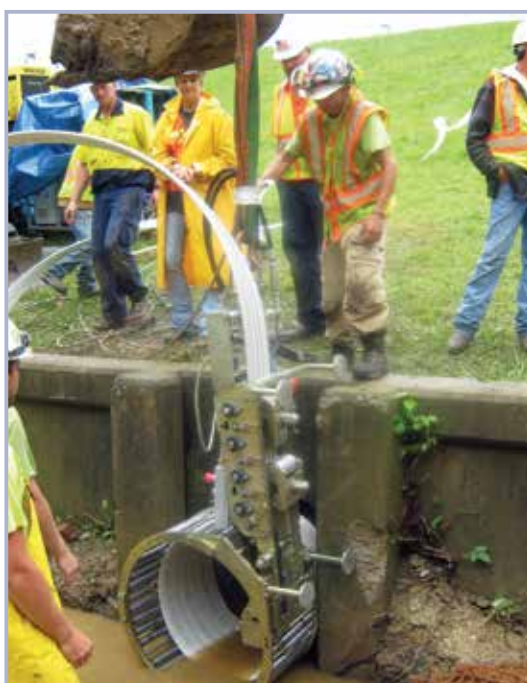
Figure 10.73 Typical installation of a spiral wound pipe liner, Jeffersonville/Clarksville Levee System in Indiana, USA (courtesy Christina Neutz)
