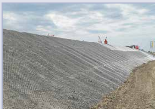
Figure 10.31 Installation of protection grid on the levee (courtesy EGIS)
