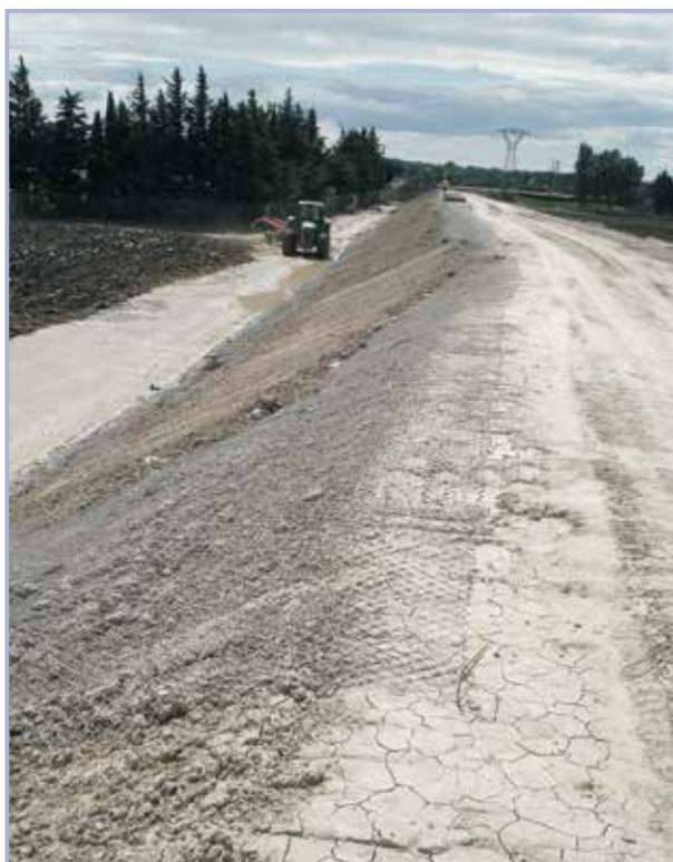
Figure 4.33 Metal mesh on the surface of the levee (courtesy Symadrem)
