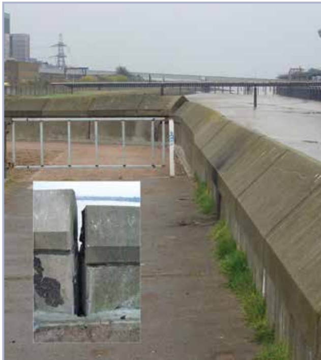
Figure 9.148 Differential movement between pre-cast crest wall units (courtesy Mike Wallis)
