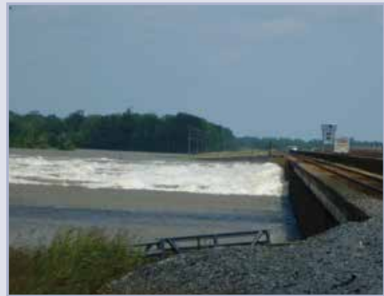
Figure 9.144 Morganza control structure discharging floodwaters during 2011 flood on Mississippi River; note the vigorous discharge (courtesy USACE New Orleans District Archives)
