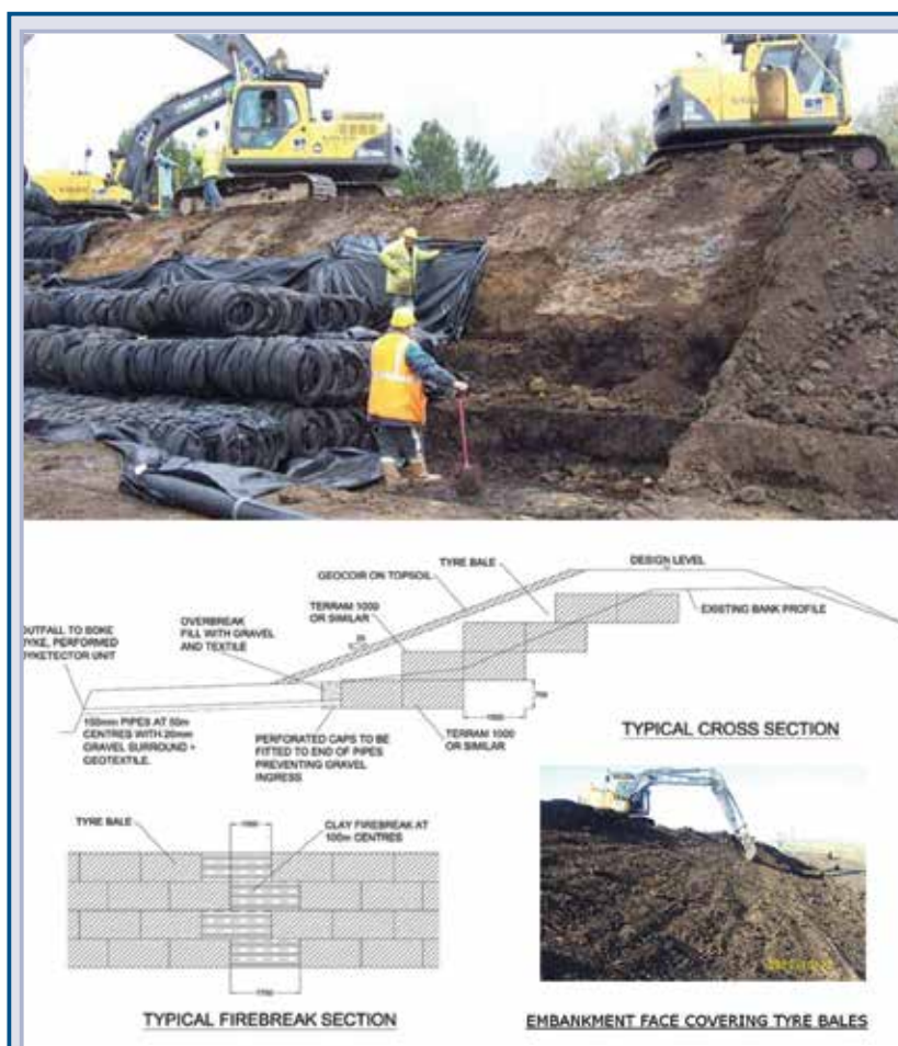
Figure 9.107 Use of tyre bales for levee rehabilitation (courtesy Environment Agency)
