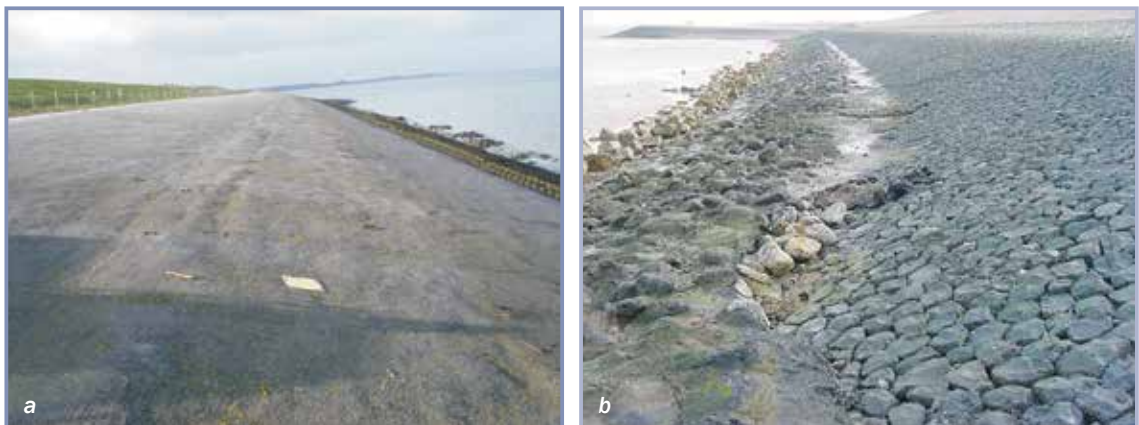
Figure 6.29 Examples of levee with asphalt (a) and stone revetment (b) (courtesy STOWA)
