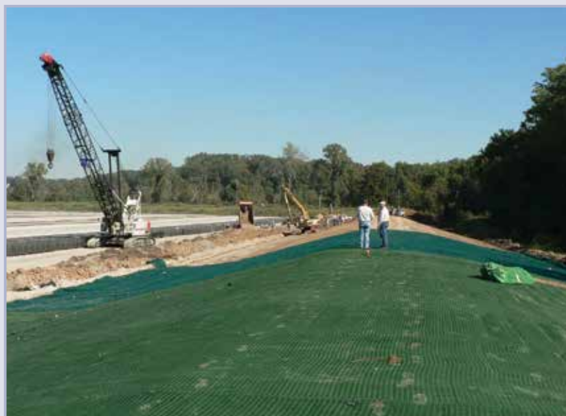
Figure 9.25 Turf reinforced mattress (from USACE, 2011)
