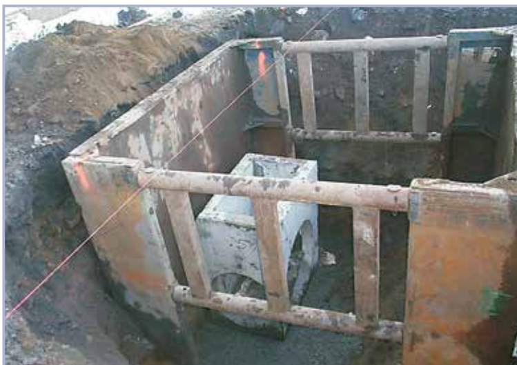
Figure 10.71 Sanitary sewer line penetration before levee construction (courtesy Lawrence Piazza)
