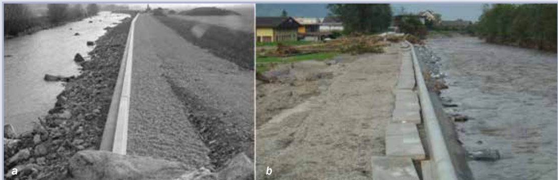
Figure 9.141 Weir fuse on the right bank of the Aa Engelberger (a) before flood, and (b) after flood (Degoutte et al, 2012)
