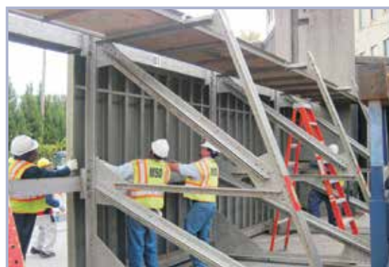
Figure 4.55 Intermediate truss supports pinned in place
