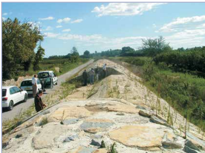
Figure 3.97 Spillway on the Vidourle River (courtesy G Degoutte, Irstea)
