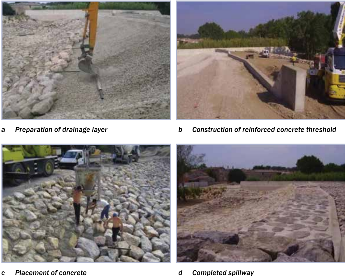
Figure 9.121 Construction of rockfill concrete spillway (Degoutte et al. , 2012)
