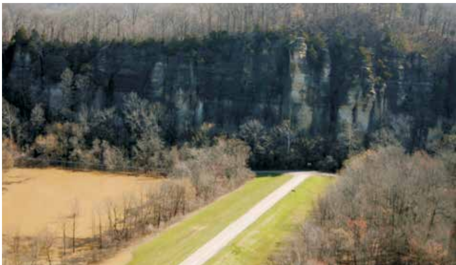
Figure 3.7 Levee abutting a natural topographic feature, southern Illinois, USA
