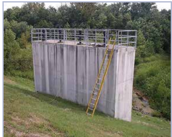
Figure 3.120 Gatewell structure (courtesy USACE)
