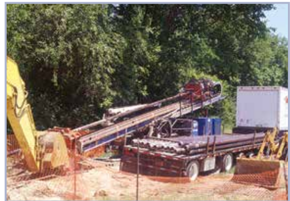
Figure 3.144 Horizontal directional drilling rig (courtesy USACE)
