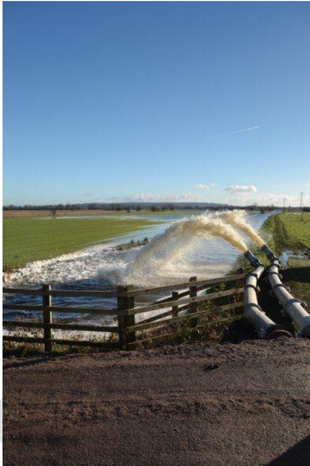
Figure 8 Pumping flood water on the Somerset Levels and Moors, South West England, winter 2013/14
