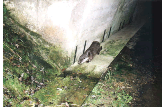
Figure 7.62 - A board placed inside the culvert is regularly used by otters in this Czech culvert. (Photo by V. Hlaváč)
