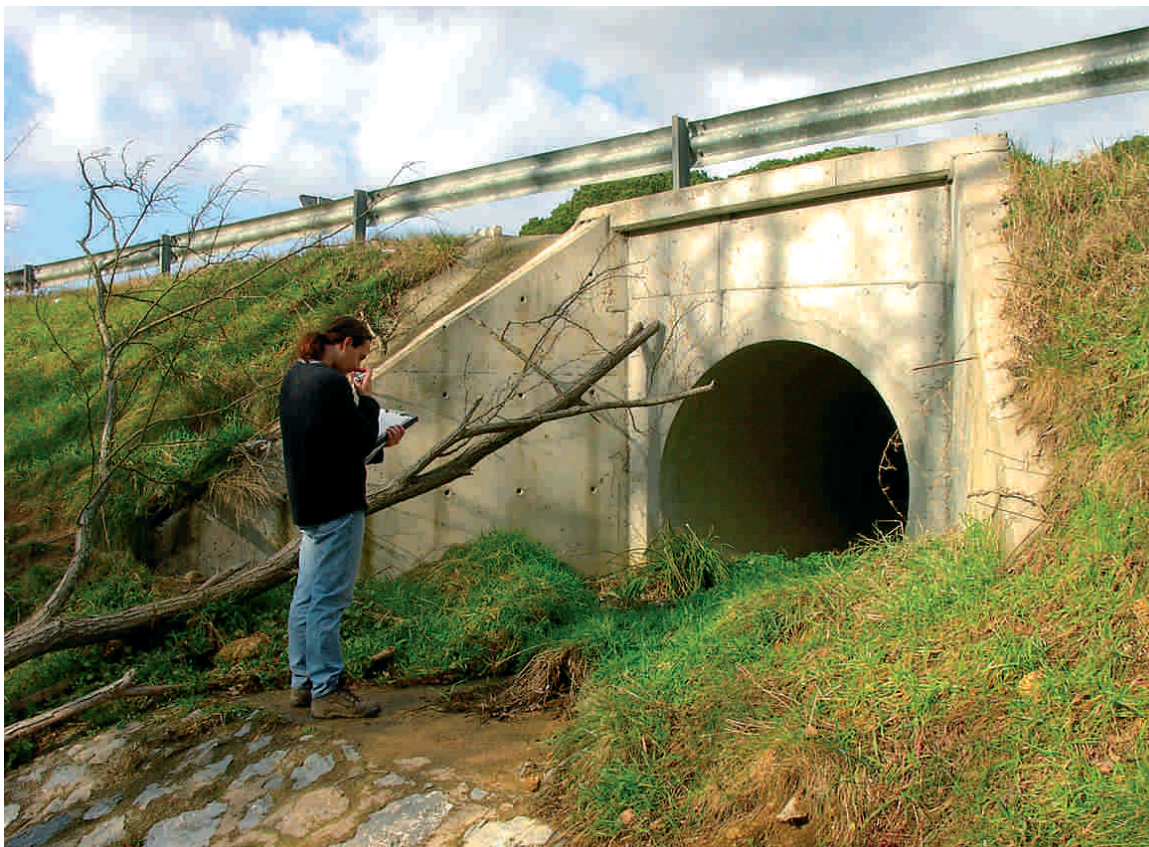
Figure 9.1 - Monitoring of fauna passages or registering road casualties to locate black spots can be carried out by standard procedures included in the infrastructure maintenance plans. (Photo by C. Rosell)
