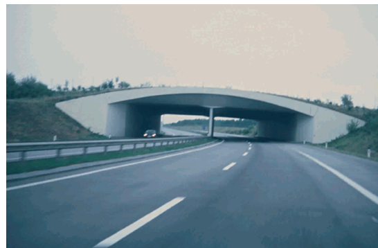
Figure 7.23 - A wildlife overpass east of Vienna (Austria), one of five in a row across the A4. (Photo by H. Bekker)
