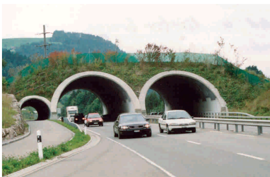
Figure 7.24 - This picture shows the same overpass Schindellegi as in figure 7.22 after it was finished. The slope on the right-hand side is very steep, but as the overpass lies on a mountain slope, red deer and other animals use it frequently. (Photo by V. Hlaváč)
