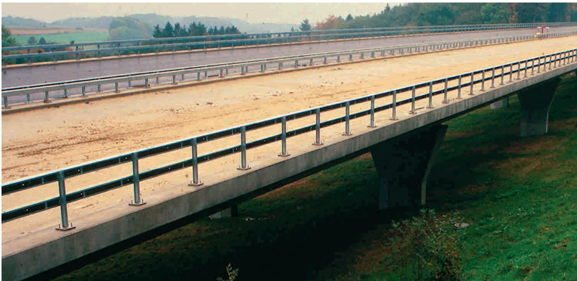
Figure 7.37 - A long viaduct on a slope as opposed to an embankment preserves the habitat and allows animals to move freely, as with this example of a Swiss motorway. (Photo by H. Bekker)
