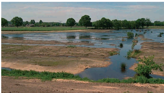
Figure 8.1 - Mosbulten (NL). Above: to compensate for the loss of marshland habitat due to the construction of Highway A50 Eindhoven-Oss, the first thing to do was transform set-aside farmland by removing the top soil. Below: after removal of the soil of former arable land, marshland habitat may develop and attract breeding birds. Target species are reed warbler and water rail. (Photos by H. Bekker)
