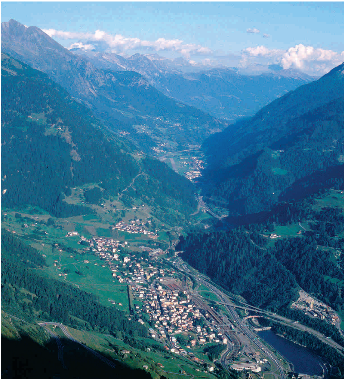
Figure 3.1 - In valleys such as in the Valle Leventina in the Swiss alps railway lines, motorways and other roads often lie close together at the valley bottom. Together they form strong barriers. (Photo by V. Keller)
