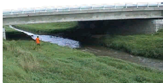
Figure 7.48 - If bridges over streams are built wide enough to preserve the natural banks of the river, they can be used as underpasses by animals, like in this example from the Czech Republic. (Photo by J. Dufek)
