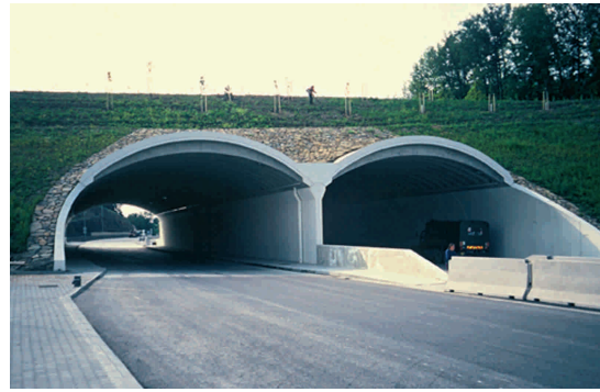
Figure 7.21 - Wildlife overpass in the Czech Republic with two prefabricated arches made of concrete. (Photo by H. Bekker)
