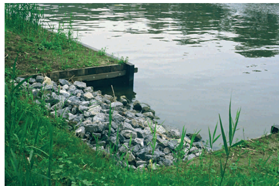
Figure 7.96 - Different possibilities for fauna exits on waterways in the Netherlands. Exits at the water side of the sheet piling is only possible when there is no danger for ships. In use by badgers, roe deer, young ducks and hedgehogs. (Photos by H. Bekker)
