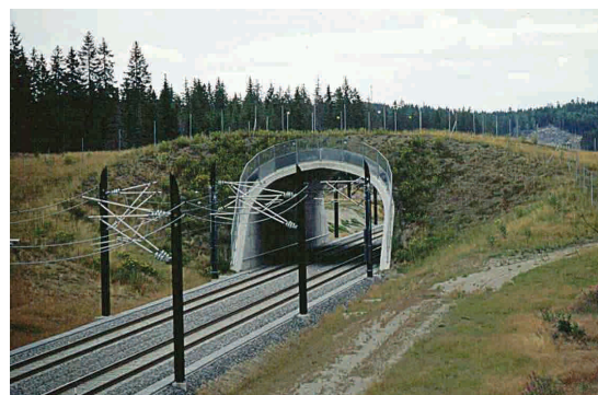
Figure 7.25 - A wildlife overpass across a high-speed railway line in Norway (44 m wide) preserving an important migration route of moose. (Photo by L. Kastdalen)
