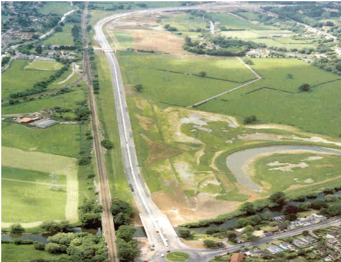
Figure 6.1 - A4/A46 Batheaston/Swainswick bypass - within the Cotswolds Area of Outstanding Natural Beauty (AONB) and adjacent to the World Heritage City of Bath, UK. Landscaping was developed with highway design to ensure the best possible fit with the landform. There was extensive use of false cuttings and shallow embankments to screen traffic and blend the engineering slopes gently into the landform. (Photo by Highways Agency, UK)
