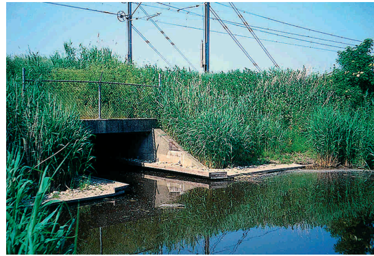
Figure 7.63 - An adapted culvert under a railway in the Netherlands. The ledge needs a good connection with the embankment, a width greater than 0.7 m and to be made of concrete, stone or wood. The design should be as open as possible. (Photo by H. Bekker)
