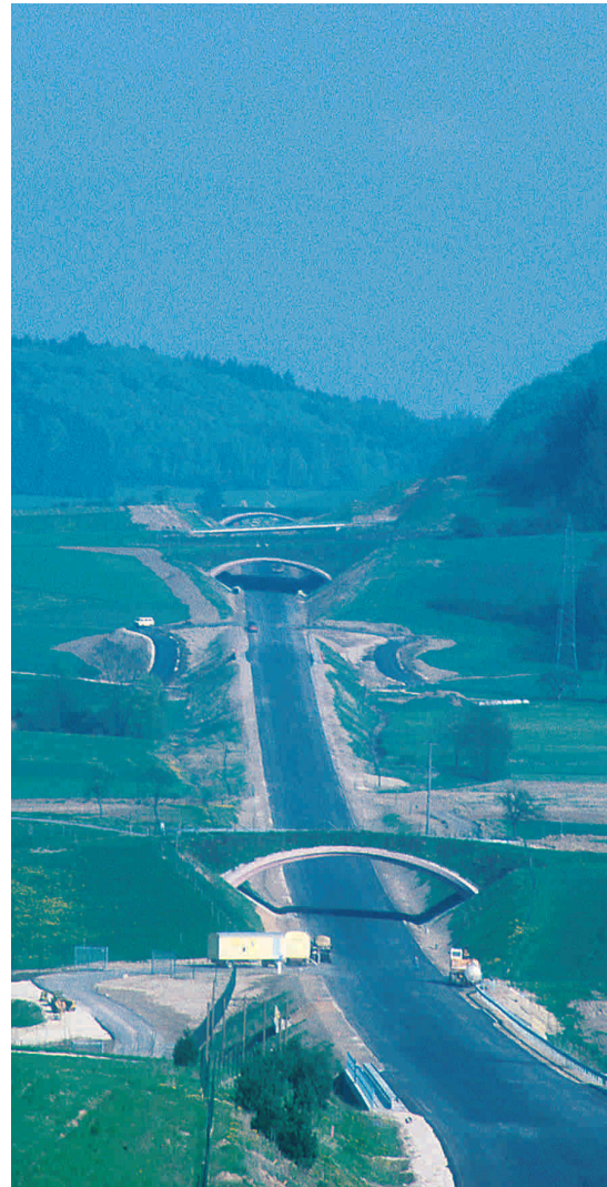
Figure 7.7 - The three-lane highway B31n in Southern Germany cuts off an area along Lake Constance. A high density of passages prevents the habitats from becoming isolated. Passages include wide wildlife overpasses as well as narrower ones combined with agricultural and forestry tracks. (Photo by V. Keller)
