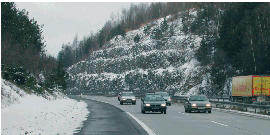
Figure 6.8 - Terracing breaks up deep cuttings and creates new micro-habitats for a range of flora and fauna, as illustrated here on the highway D1, Czech Republic. (Photo by V. Hlaváč)
