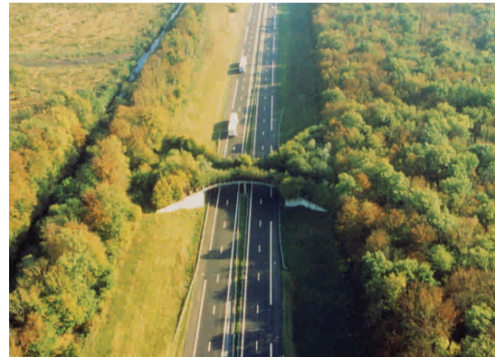
Figure 1.2 - Habitat fragmentation can be mitigated by building fauna passages like this overpass on the A36 motorway, Alsace, France. (Photo by J.Carsignol)
