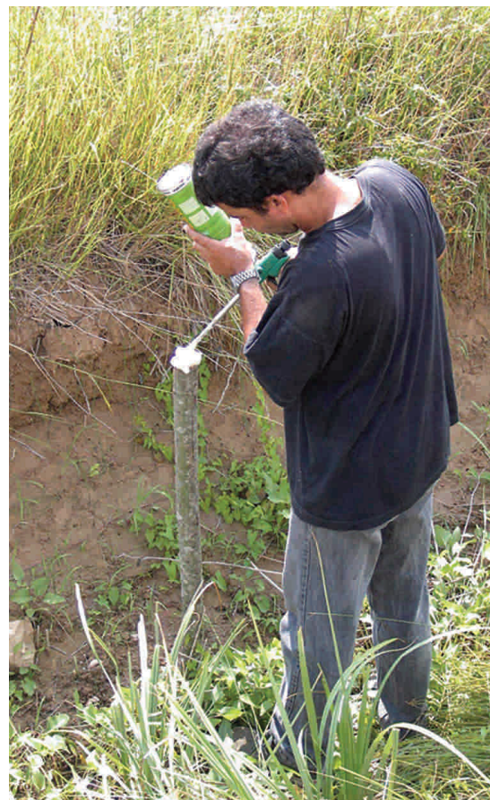
Figure 7.86 - Olfactory repellents are applied to poles along the road. (Photo by C. Rosell)
