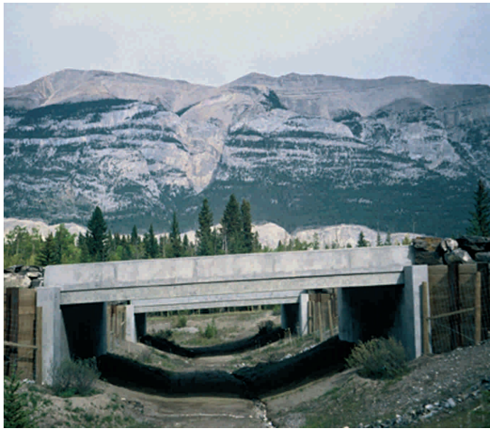
Figure 7.41 - In Banff National Park (Canada) two parallel structures were constructed to minimise the length of the underpass and to provide increased light below. (Photo by H. Bekker)
