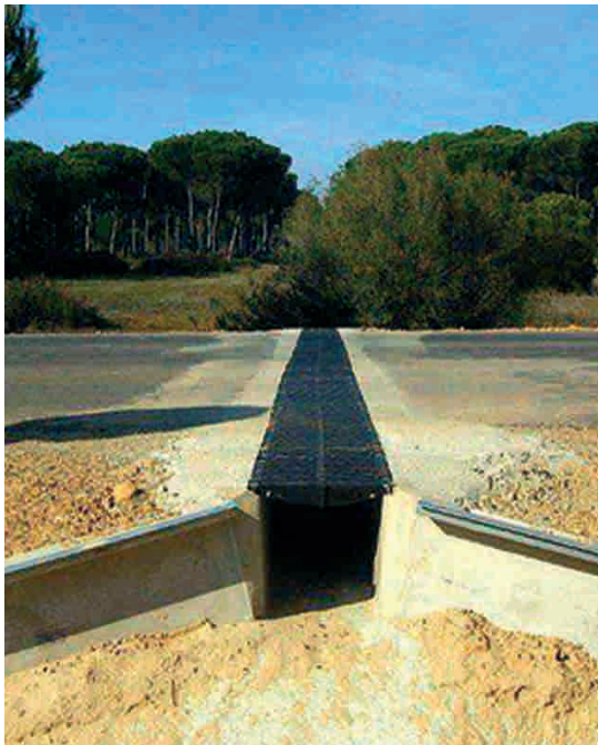
Figure 7.74 - Amphibian tunnel with open grid in Spain. (Photo by Giasa, Spain)
