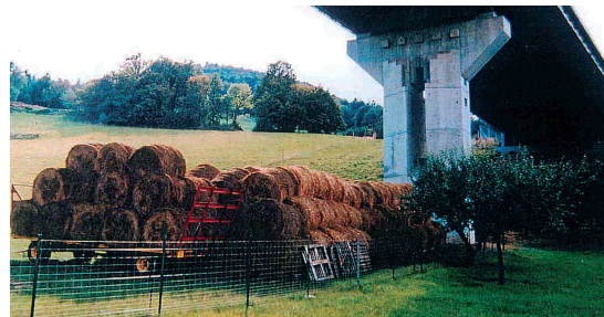
Figure 7.40 - In this example of the RN59 in France, the function of a viaduct to preserve movement of animals is lost, since access is blocked both by a fence and by stored material. (Photo by J. Carsignol)
