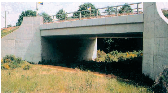
Figure 7.45 - This underpass is below a high-speed railway line in France and has a good openness index, suitable for large mammals. (Photo by SETRA)
