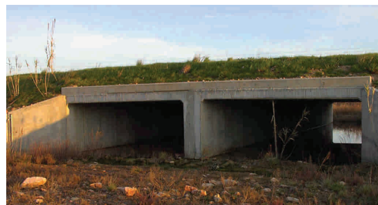
Figure 7.46 - This passage under a road which crosses a protected wetland in Spain (Natural Park Aiguamolls de l'Empordà) was constructed with a dividing wall to reduce costs: Dimensions of each section: 10 m wide (5 m each section), 2 m high, 28 m long. It is used by mammals, e.g. otter, polecat, badger and wild boar, but also by some birds from the adjacent wetland. (Photo by C. Rosell)
