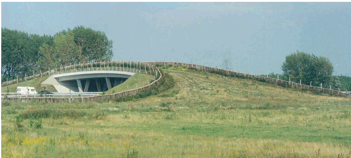
Figure 7.15 - In this example from Hungary the motorway was not cut into the surroundings. The access had therefore to be levelled out. The fences guide animals along the road verges to the overpass. (Photo by P. Farkas)
