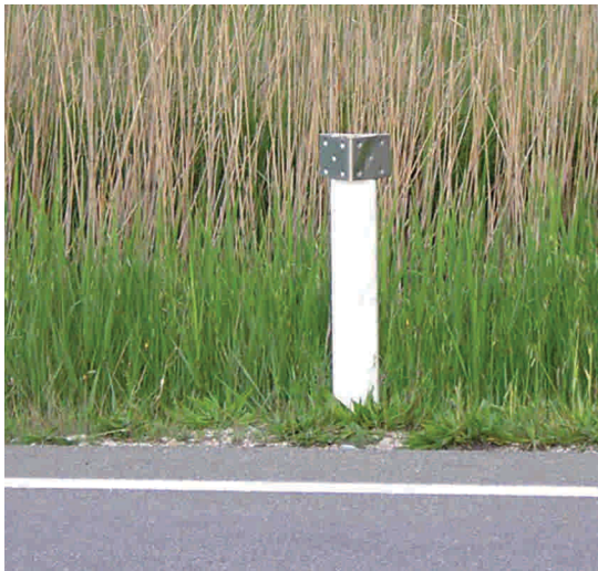
Figure 7.85 - A wildlife warning reflector in Spain. There is little evidence of the effectiveness of this measure. (Photo by C. Rosell)
