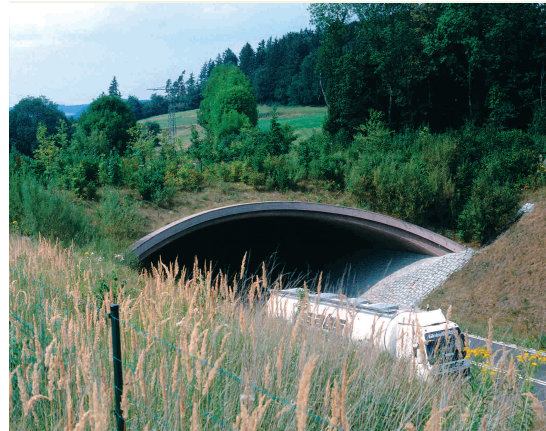
Figure 7.11 - The overpass Schwarzgraben in southern Germany (B31neu, 50 m wide, combined with local road) is densely covered with bushes and small trees since it aims at connecting the adjacent forests. (Photo by V. Keller)
