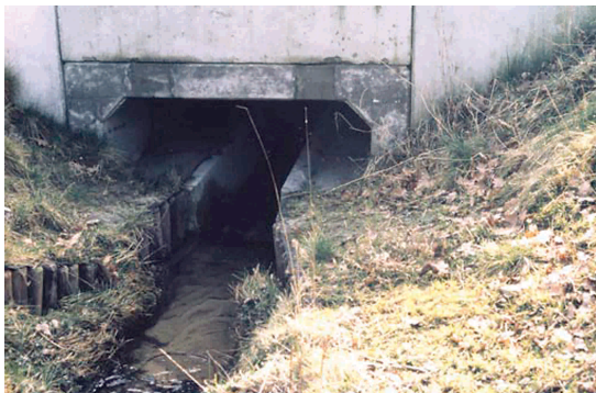
Figure 7.60 - Two prefabricated culverts in the Netherlands (A35, A1) with integrated ledges used by small animals. (Photos by G. Veenbaas and H. Bekker)
