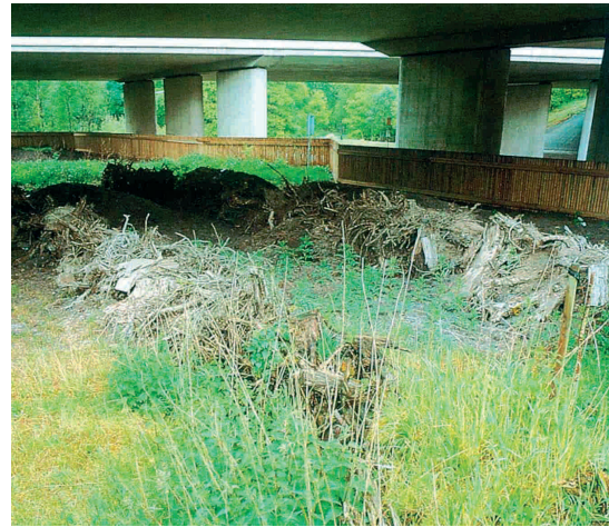
Figure 7.42 - Tree stumps were used as shelter for animals under the Zandheugel viaduct on the A27 in the Netherlands. The screen which separates the road from the stump walls can be seen in the background. (Photo by H. Bekker)
