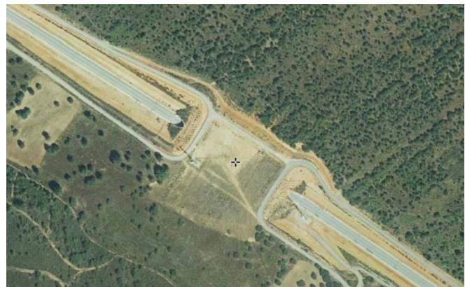
Satellite image of the viaduct. Source: iberpix, IGN
